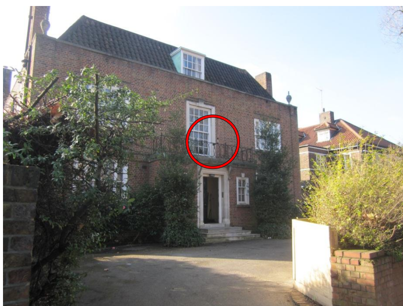
Figure 5 – Unattended Front Façade Noise Survey Measurement Position
