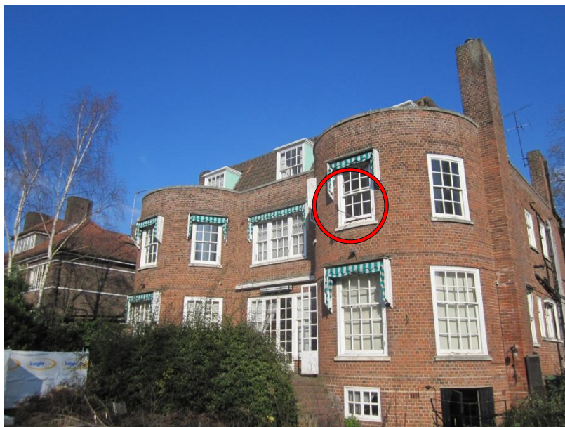
Figure 6 – Unattended Rear Façade Noise Survey Measurement Position
