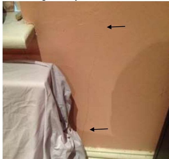
Cracking below window to bedroom
