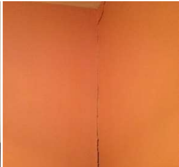
Cracking to wall junction in bedroom
