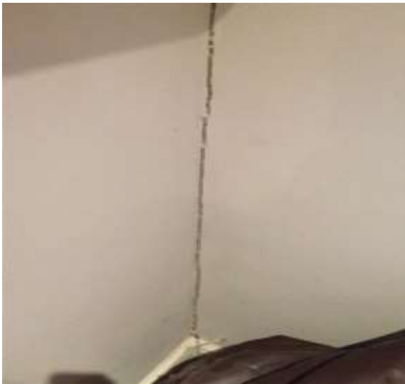
Cracking to wall junction in lounge
