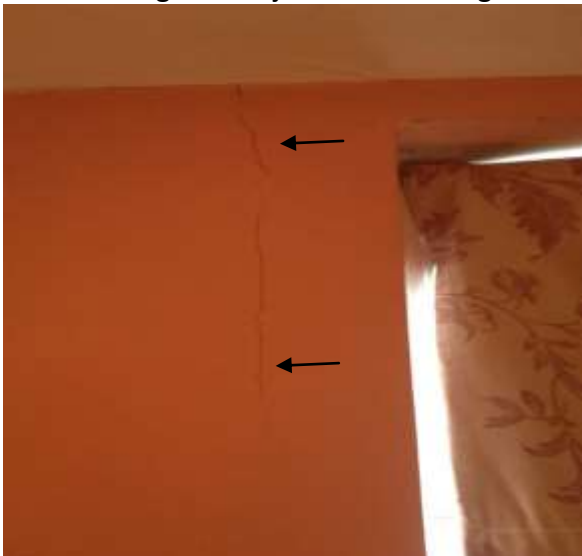
Cracking above window to bedroom
