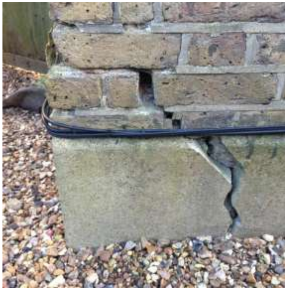
Cracking to front left corner
