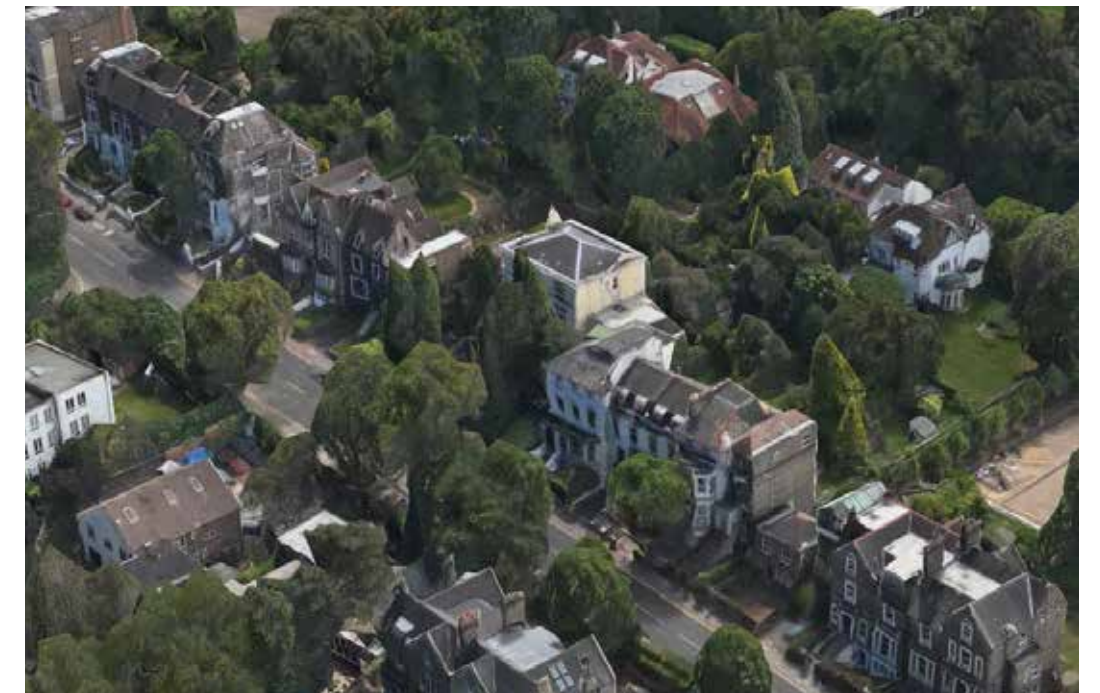
Aerial View of Roof Scape of Houses on the South Side of Hampstead Lane
