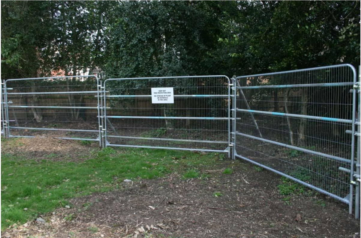
Figure 1: An example of protective fencing erected to the correct specification
