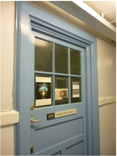
Photo of typical Type A door
