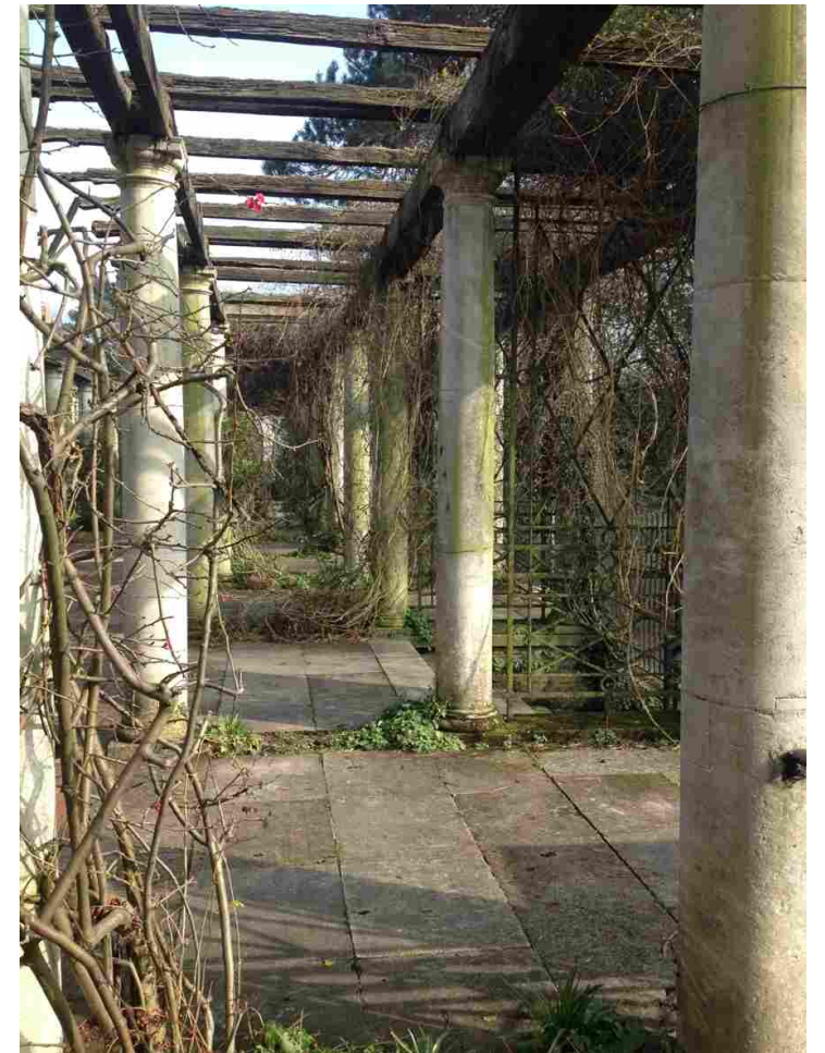
Photo of Colonnade oak timber frame looking East
