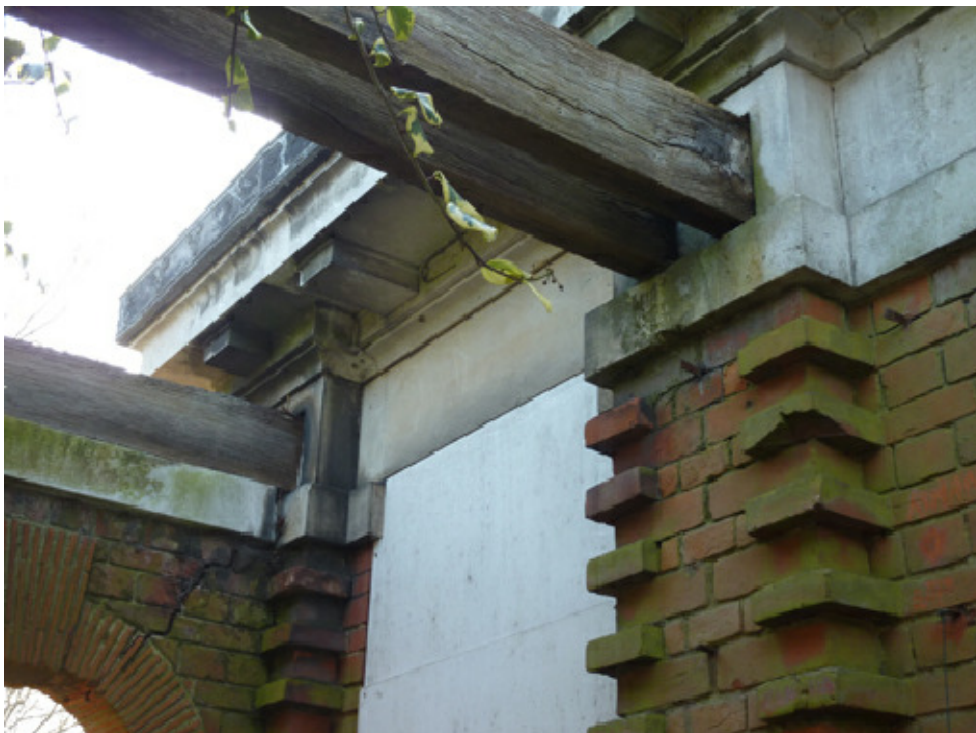
PHOTO OF CONNECTION OF PRIMARY TIMBER BEAMS TO BELVEDERE WALL DETAIL 7
