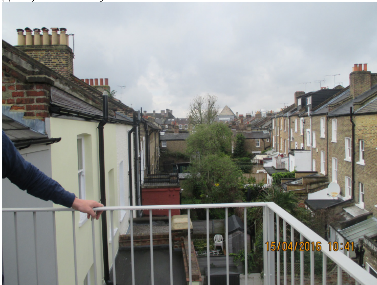
(4) Existing railings, parapet and zinc roof.
