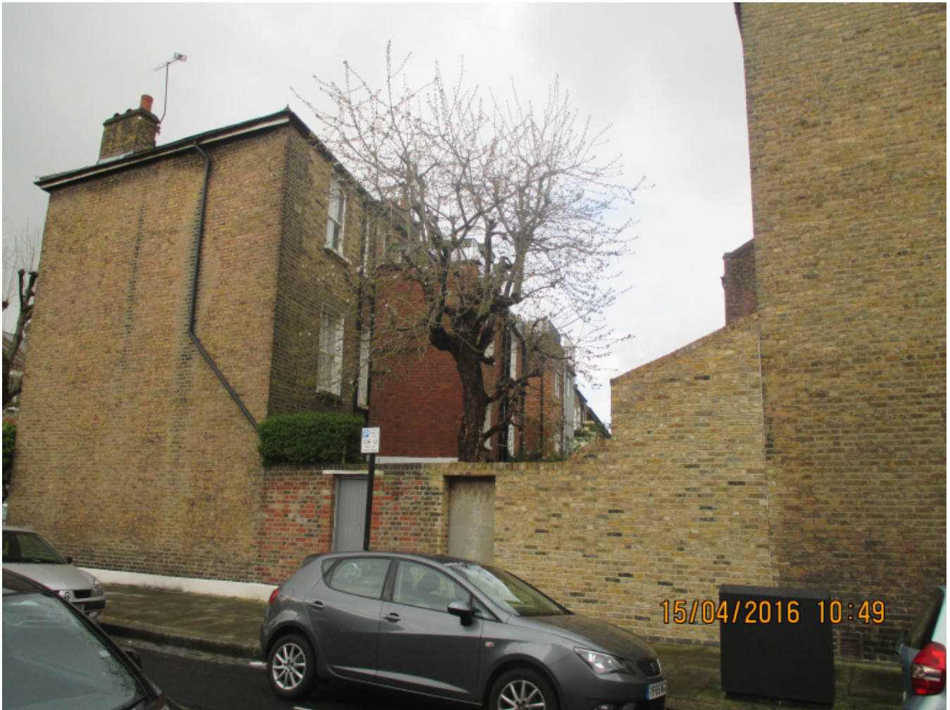
(6) View from neighbouring terrace
