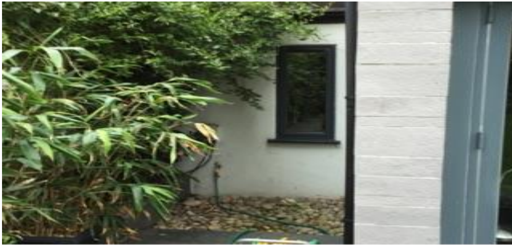
Image 3 Existing side extension
