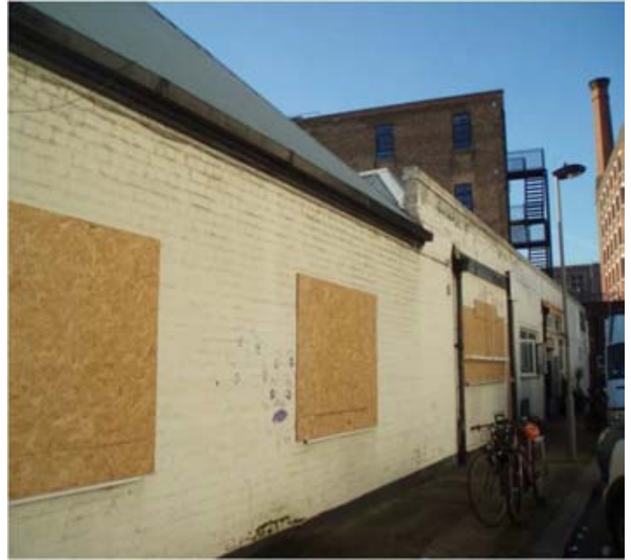
Image 10: Front of Disused Section of Greenwood Place
