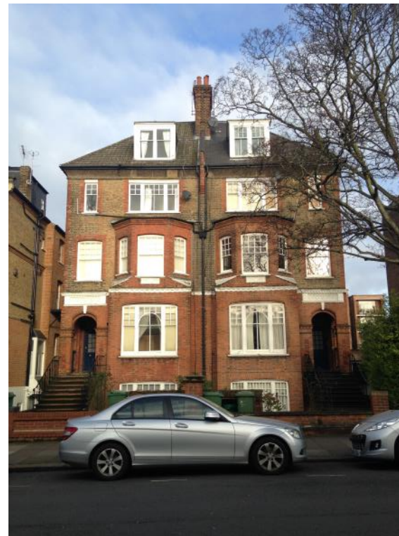
Figure 16: Main (south) façade of Nos. 86 (right) and 88 (left) Fellows Road.
