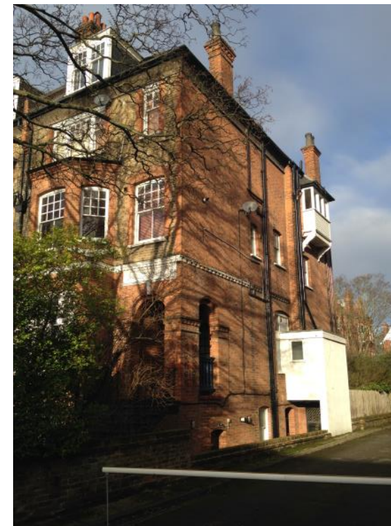
Figure 17: The east elevation of No. 86 Fellows Road showing the modern rendered side extension.
