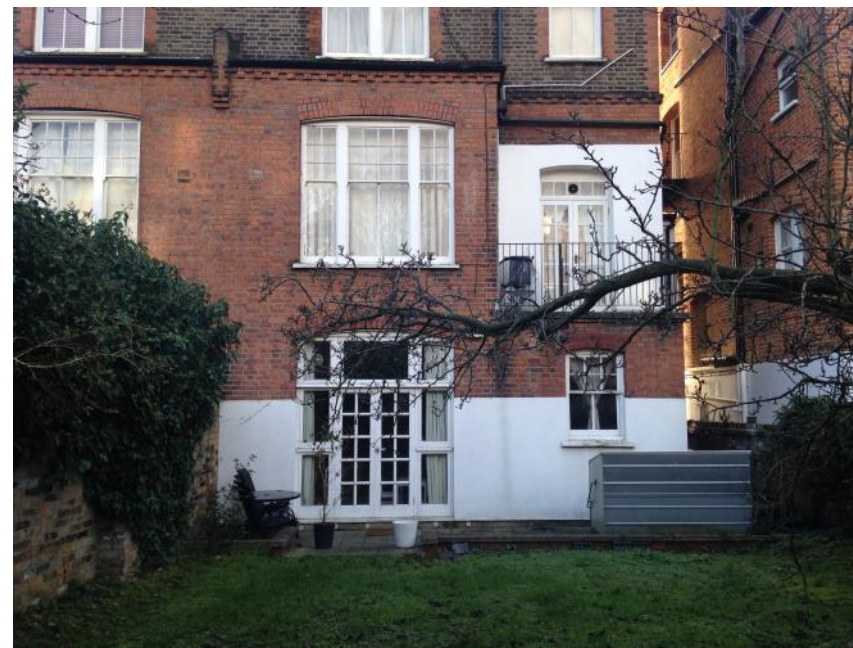
Figure 28: The rear lower and ground floor elevation of No. 88. The key differences to No. 86 are the use of render and the insertion of a door at lower ground level.
