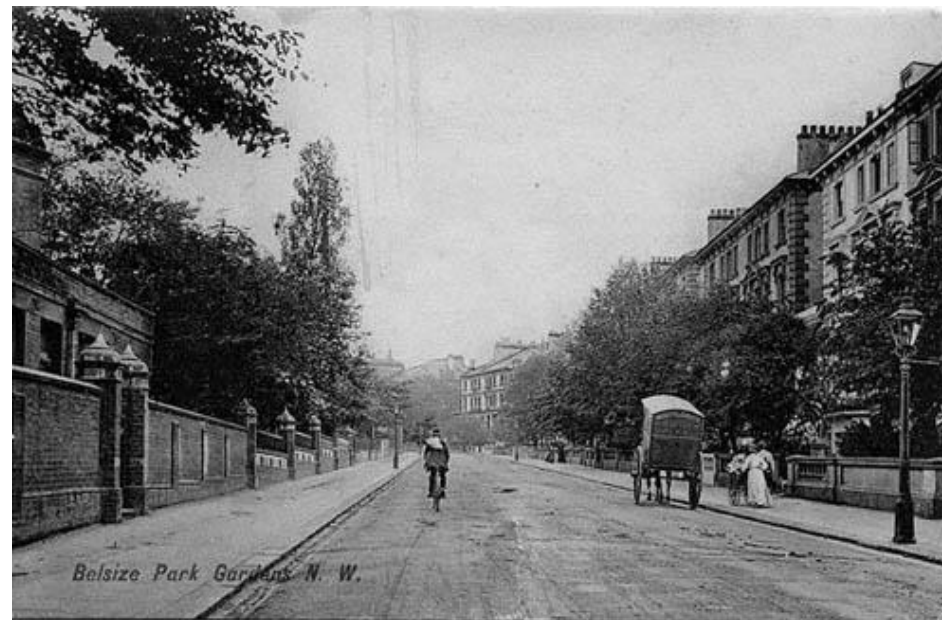
Figure 6: View along Belsize Park Gardens in 1906. This road lies to the north of the Site.
