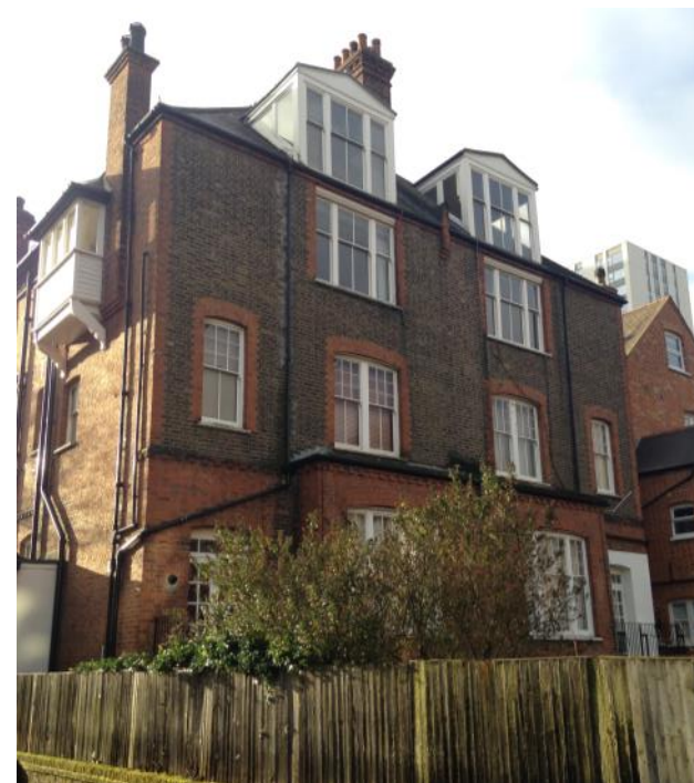
Figure 2: View of the existing rear elevation of the Site, showing the upper ground, first and second floors.
