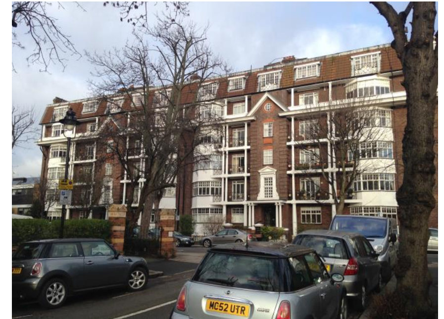
Figure 42: Eton Court, a substantial 6-storey residential block built in the late 1920s/early 1930s.
