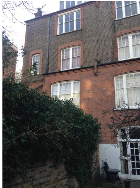
Figure 25: View of the rear elevation of the building from the garden of No. 88.
