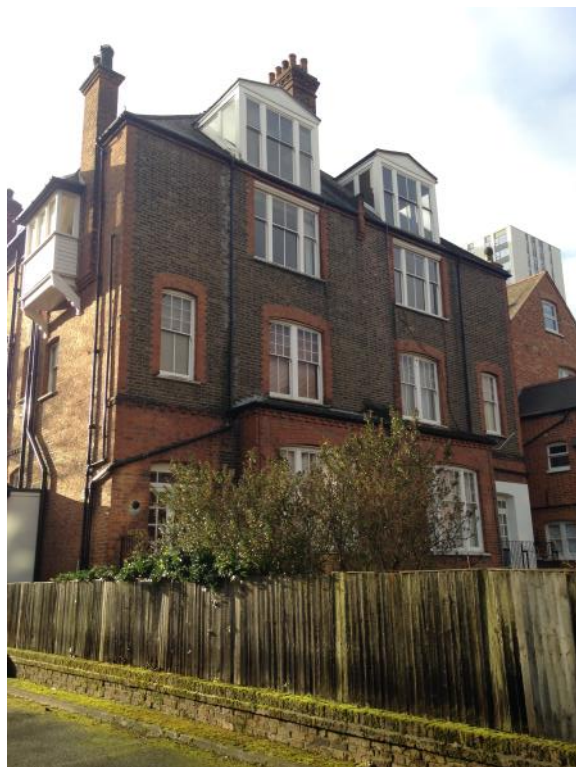
Figure 21: View of the rear elevation of the Site.
