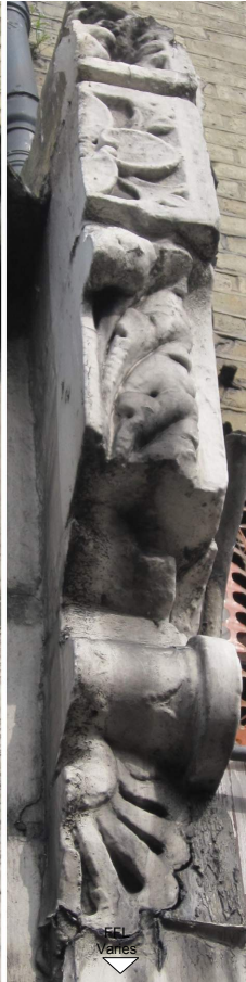
EXISTING PILASTER HEAD HALF REMOVED
