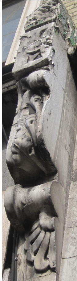
EXISTING PILASTER HEAD HALF REMOVED
