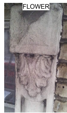
SECTION BB-FIRST FLOOR WINDOW PRE-CAST CONCRETE SURROUNDS
