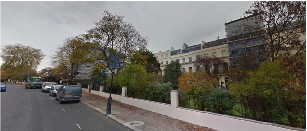
E. Property not visible from Outer Circle
