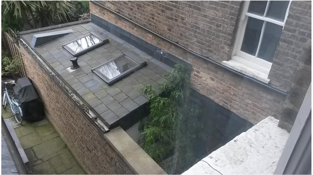
Photograph 3 : View to No.8B's lightwell from No.10.
