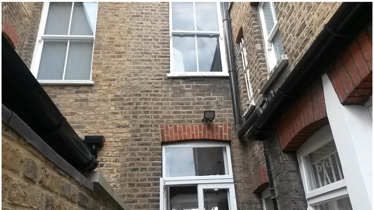
Photograph 2: Proposal area view towards the rear of No.8 and 10 Estelle Road.
