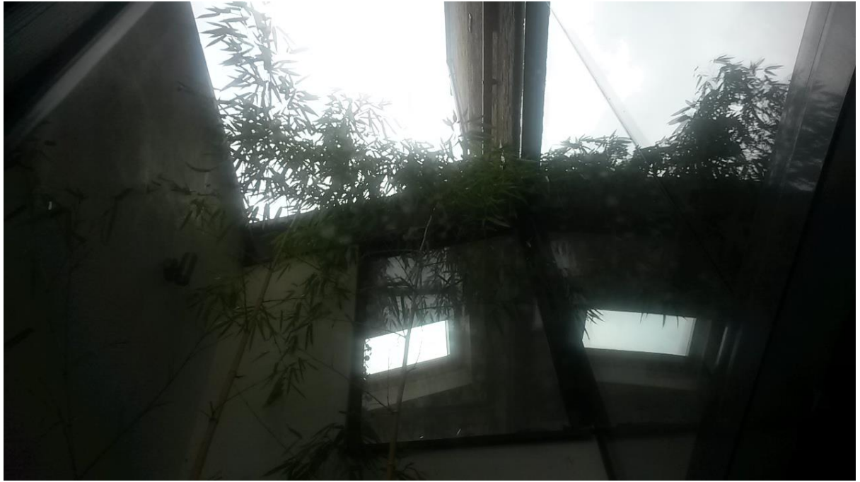
Photograph 5: View up the lightwell from No.8B basement level bedroom.
