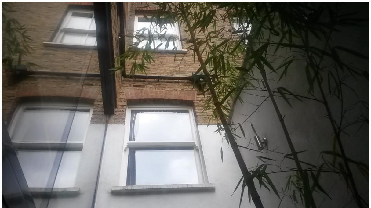
Photograph 4: View up the lightwell from No.8B basement level main bedroom.
