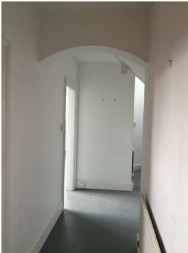
Figure 6: The archway within the hallway which has none of the proportions or detail of such features at lower levels of the building. It has the character of a later alteration.
