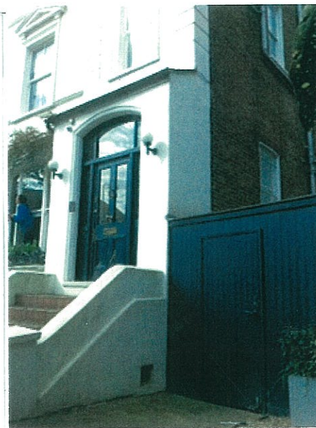
PHOTO OF FRONT ELEVATION CORNER showing 500 wd External Stone/ Render return to side elevation.
