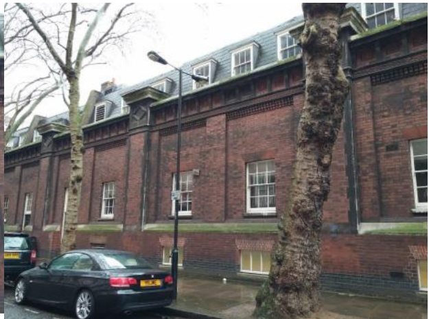
Bedford Avenue façade
