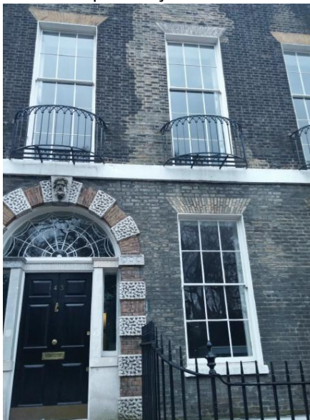
Bedford Square façade detail
