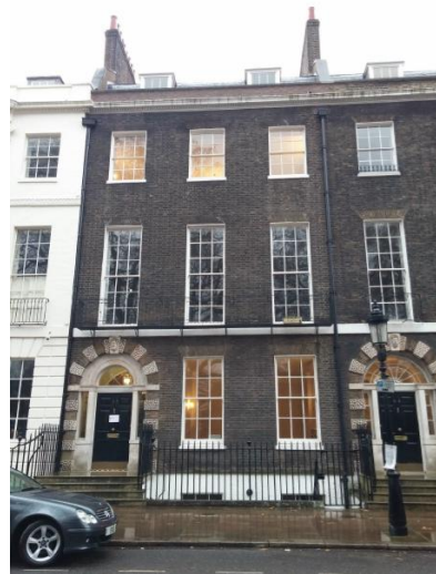
Bedford Square façade detail
