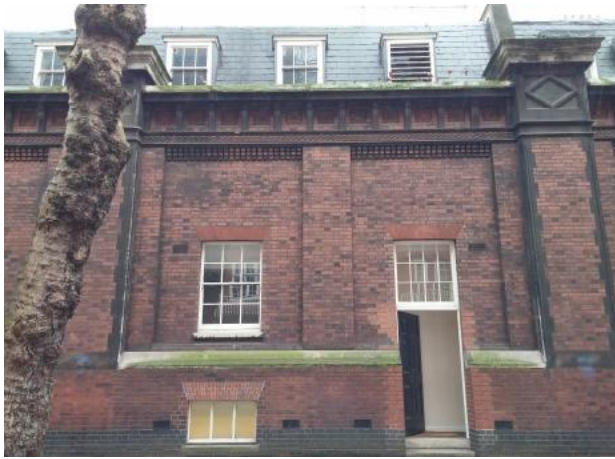
Bedford Avenue façade
