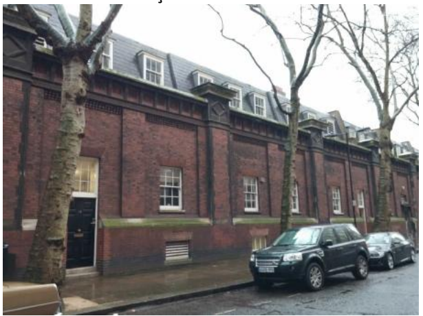
Bedford Avenue façade
