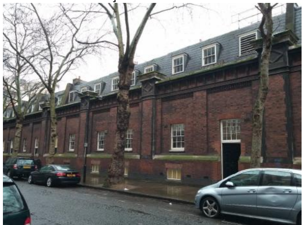
Bedford Avenue façade
