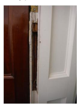
The existing frames will be repaired where damaged by previous installations, and the doors will be re-hung on new fire rated hinges.
