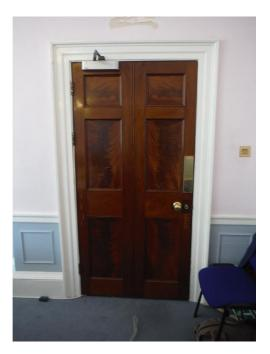
It is proposed to carefully remove and set aside the existing doors and remove the existing brass ironmongery
