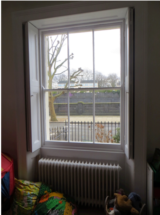
Figure 5. Photograph of ground floor front window with full length original wooden shutters.
