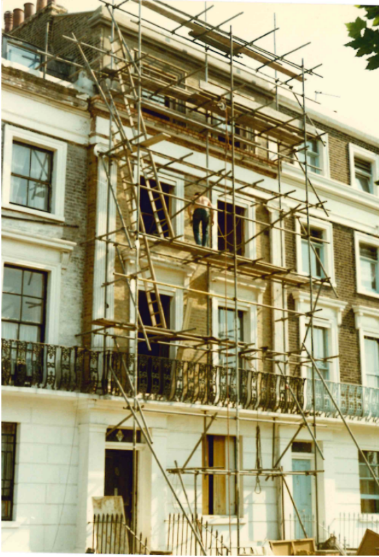
Figure 2. Photograph of window installation, taken in the Summer of 1984.
