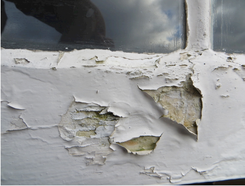
Figure 4. Photograph of front upper floor window.
