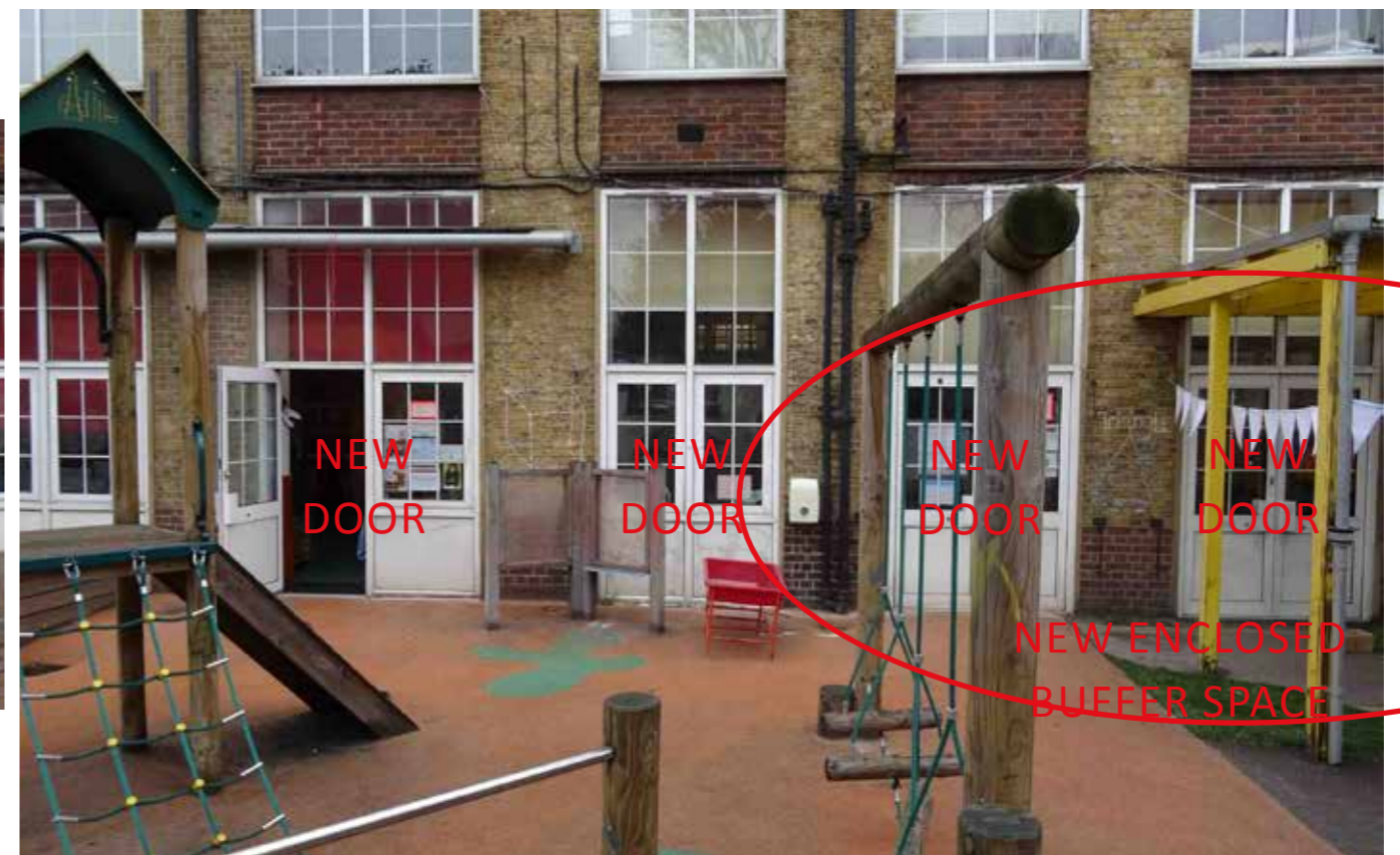
New Buffer Space to be constructed in front of 3no. existing openings. New Canopy in front of Buffer Space.
