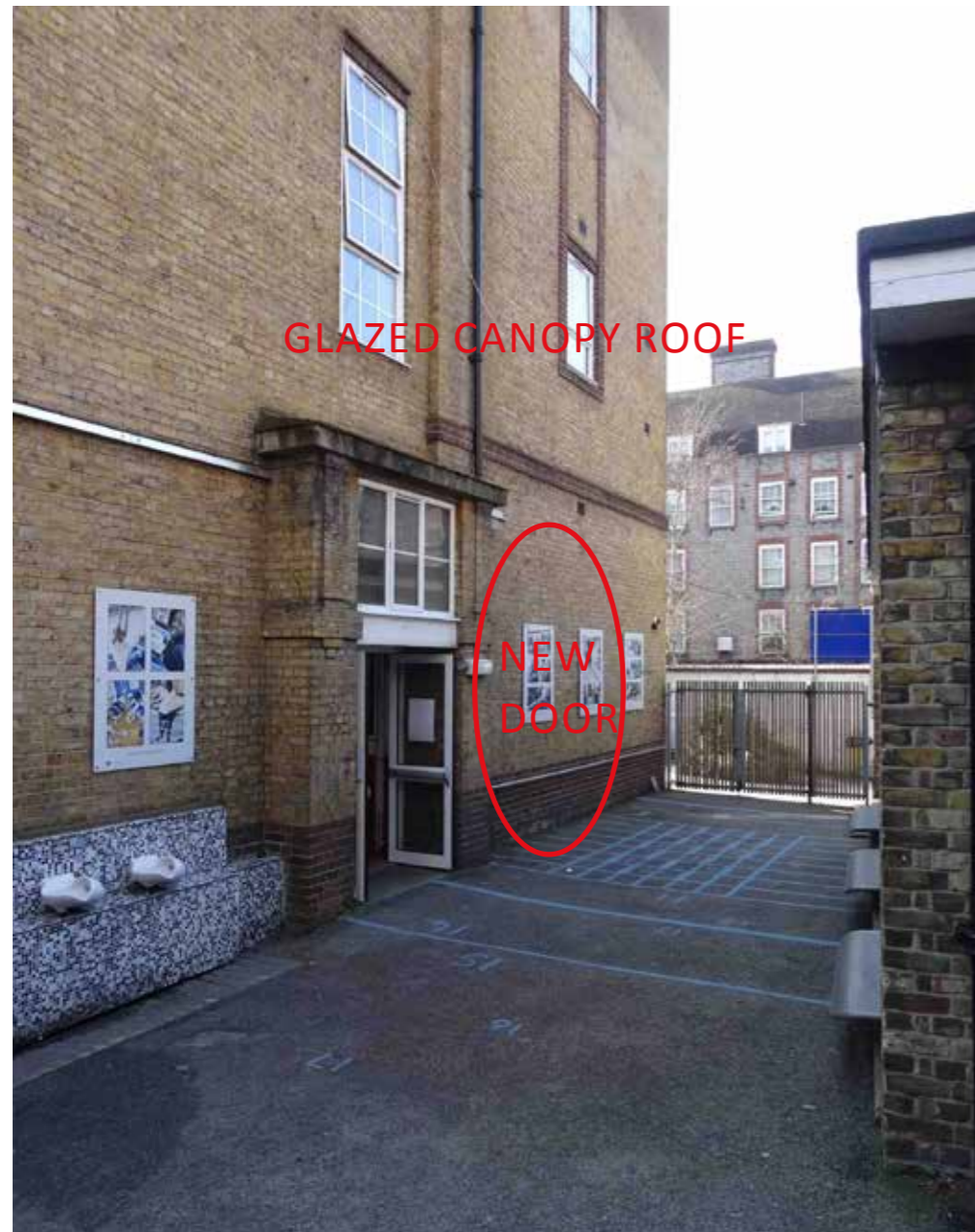
Location of proposed new entrance to the reception. A glazed canopy roof is to form a dry link between the main building and the dining room (to the right).
