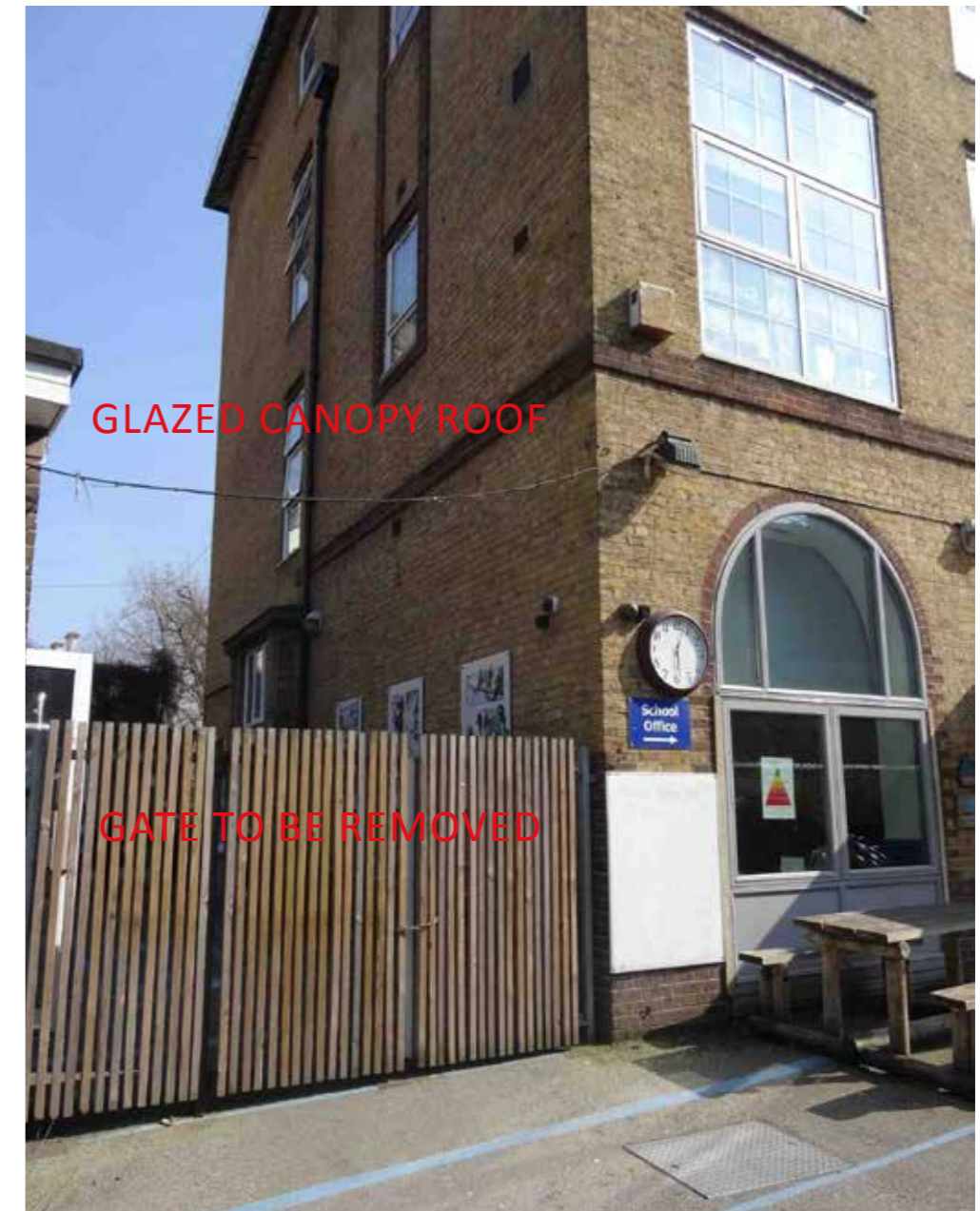
Entrance approach from Cliff Villas. The existing fence is to be removed, and a new side access formed to the reception. A glazed canopy roof is to form a dry link between the main building and the dining room (to the left).
