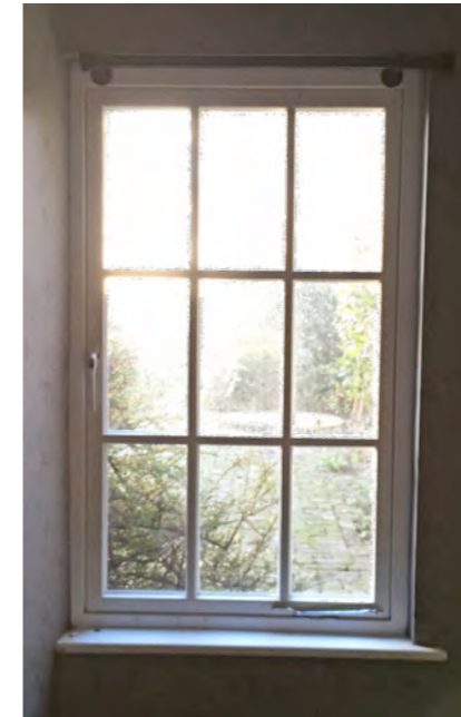
CASEMENT TO BE REPLACED
