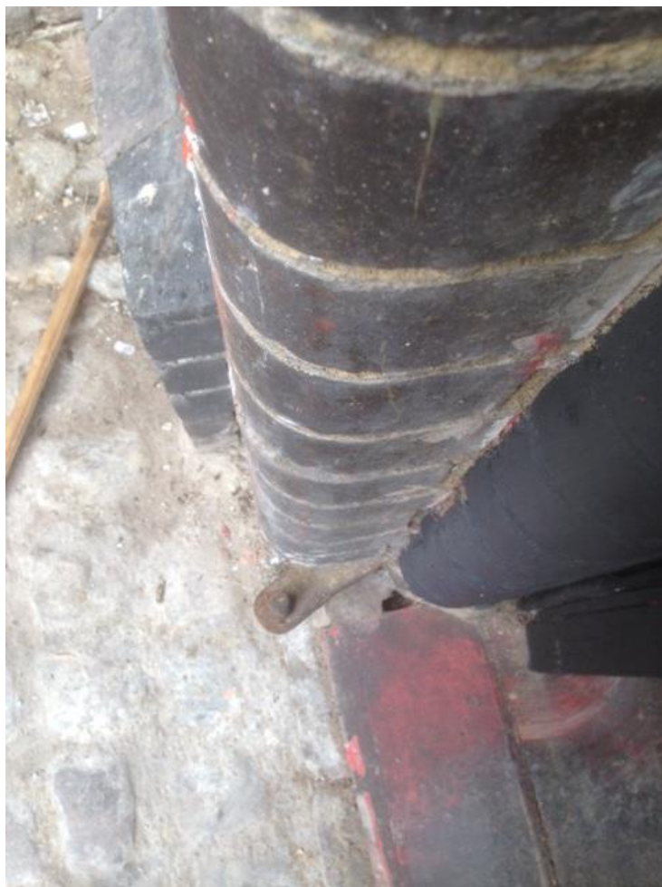
Figure 17 2016 photograph showing double bullnose reveal detail to the narrower door opening. Note the brick plinth and the remaining pintle from the original stable door.
