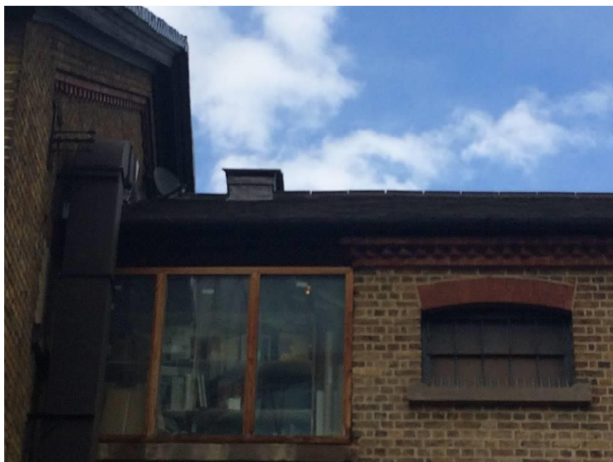
Figure 13 2016 photograph showing the extant former stable roof ridge ventilator which is to be reconstructed to serve as the extract cowl for the new extract system.
