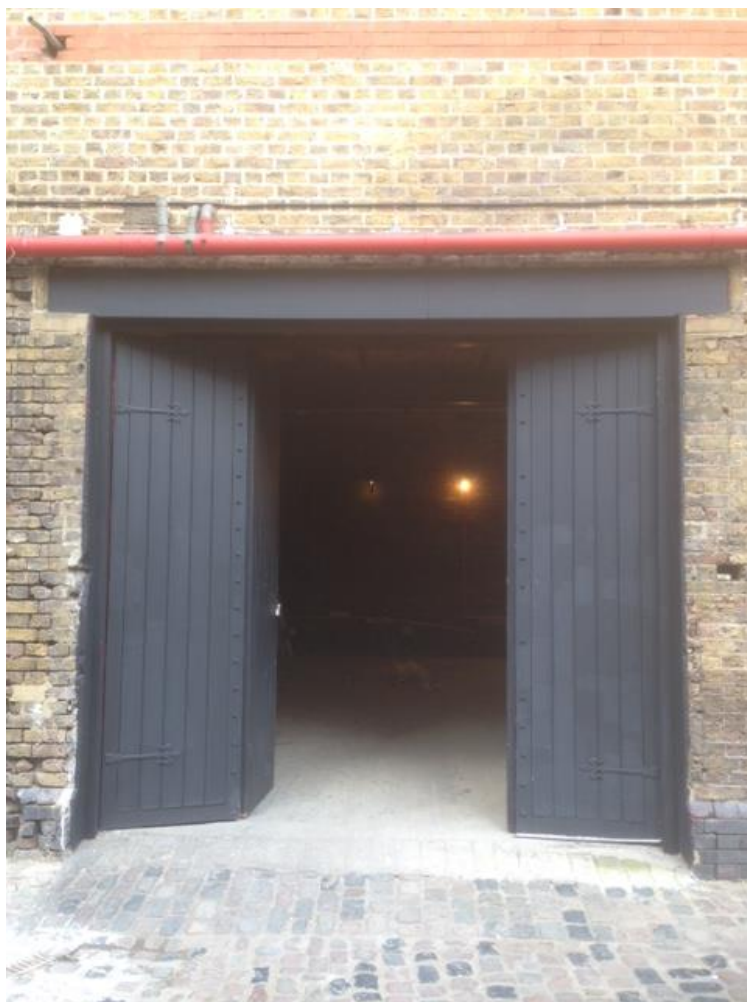
Figure 11 2016 photograph showing the later modified widened opening with steel lintel over (Unit 92).
