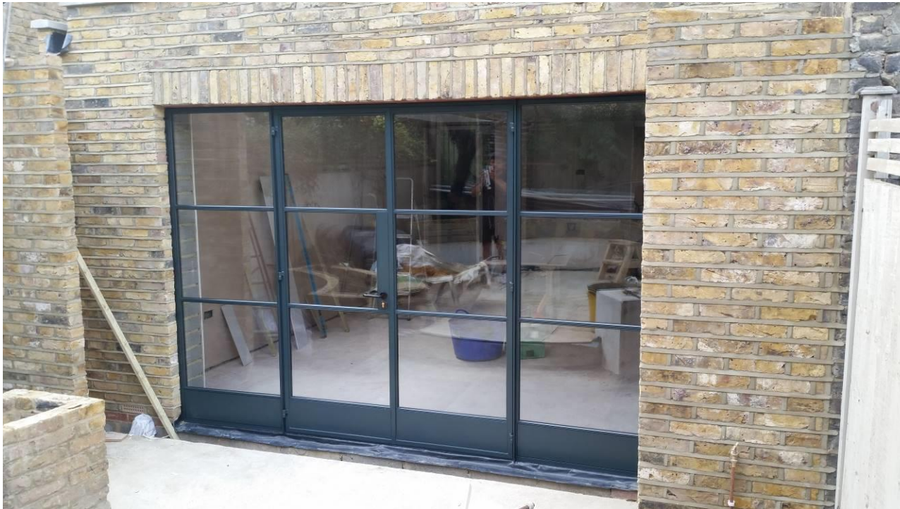
Figure 23 Typical steel framed and glazed door arrangement.
