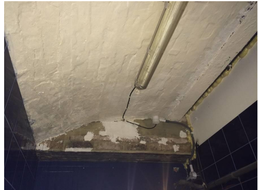
Figure 16 2016 photograph showing interior ceiling soffit in north west corner. A high level aperture above the opening will be formed through the wall to allow the routing of the supply air duct.
