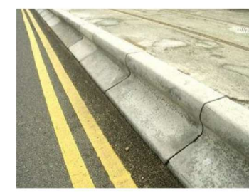
High Containment Kerb To eastern road edge
