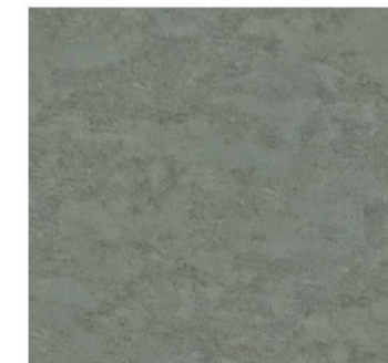
Concrete Wall In-situ concrete with waterproof additive.
