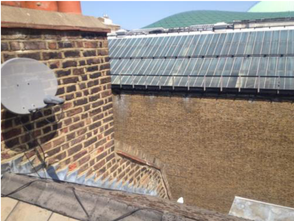
P3 General view of flank wall
