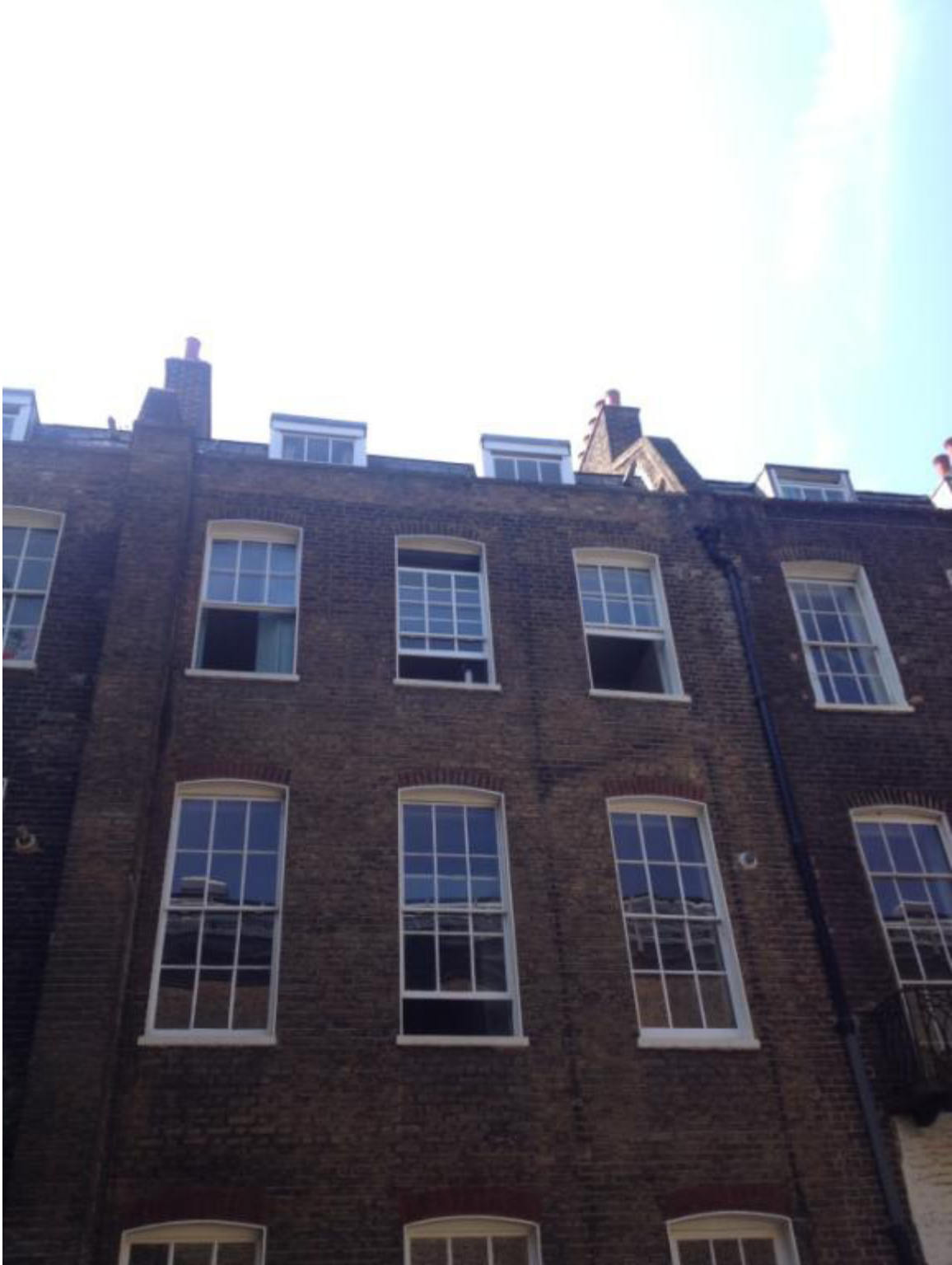
PI General view of rear elevation
