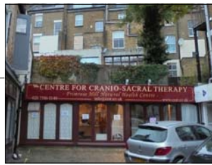
REAR FENCE AND FLAT VIEWED FROM ST. GEORGE'S MEWS
