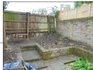
EXISTING RAISED BED AND REAR FENCE VIEWED FROM FLAT
