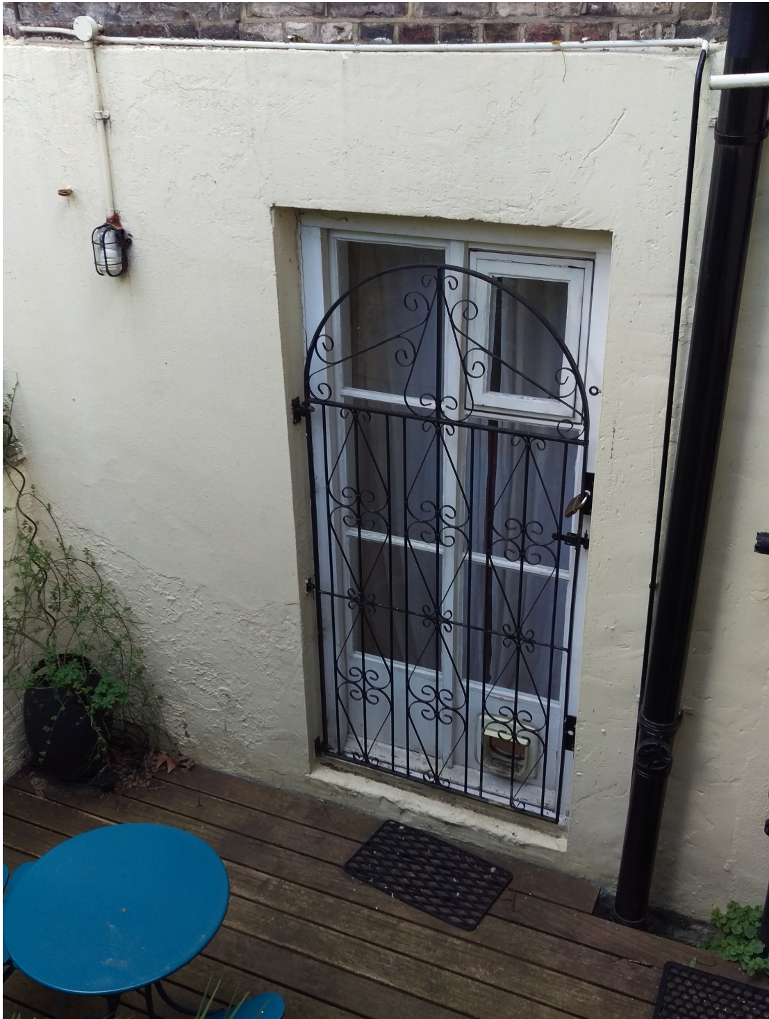
1. Window in the main bedroom changed to doors
