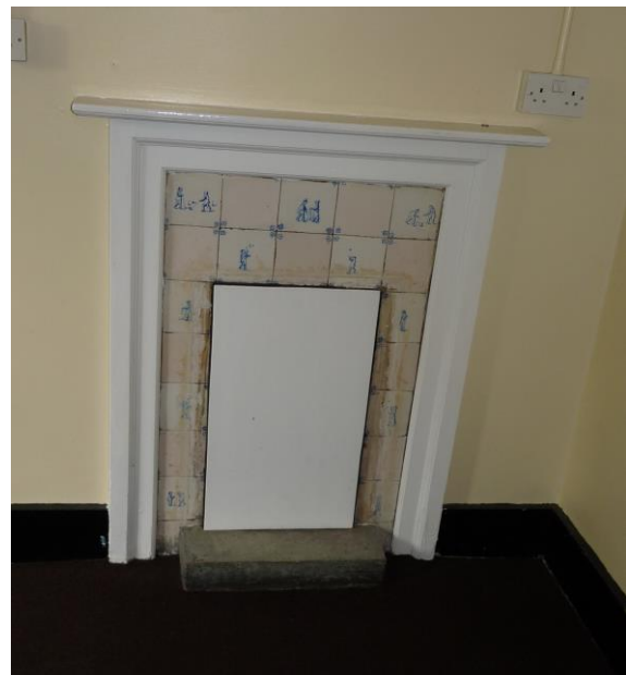
Domestic fire place
