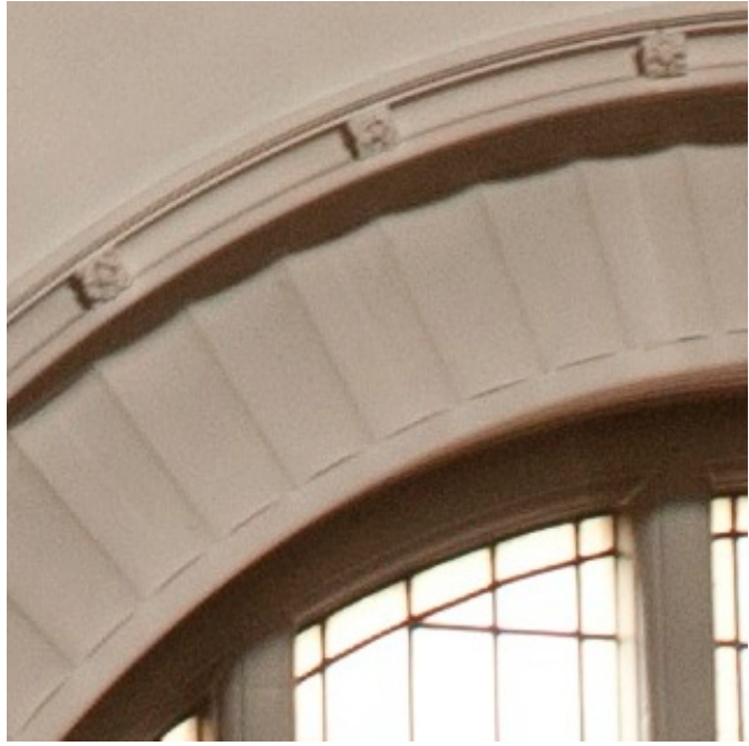
A Detail A Fluted architrave moulding - first floor chapel window
