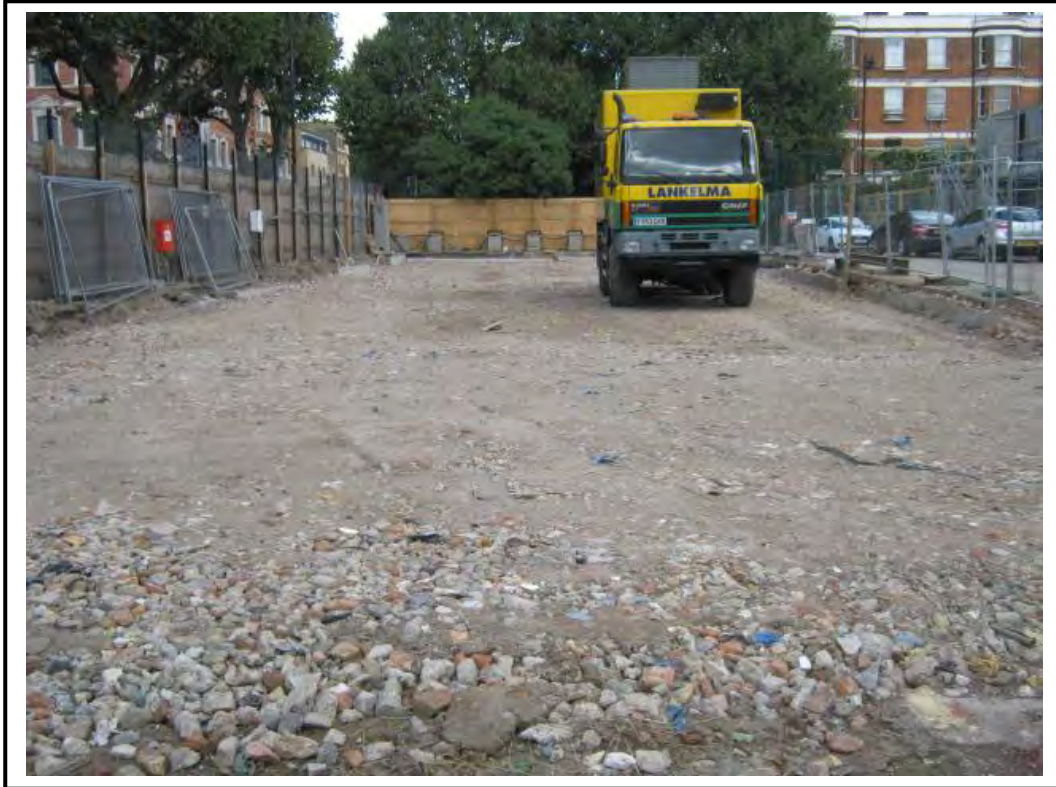
Completed piling mat undergoing geotechnical testing.
