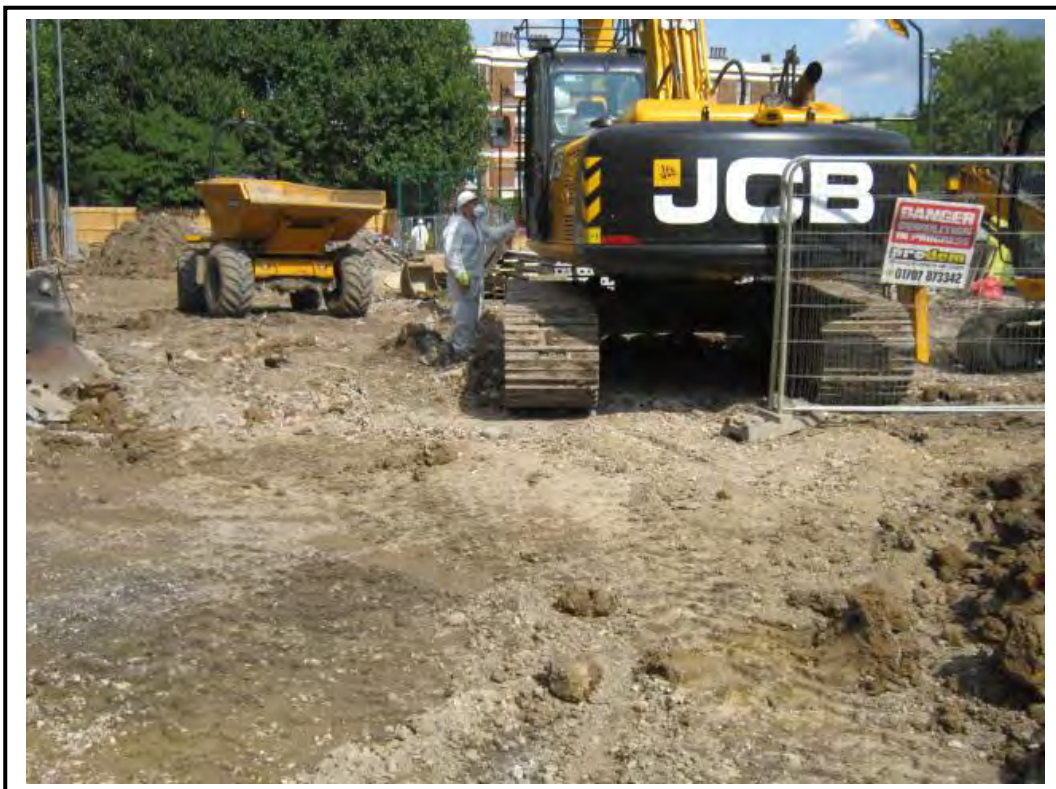
Excavation of asbestos contaminated soils with operatives in disposable overalls
