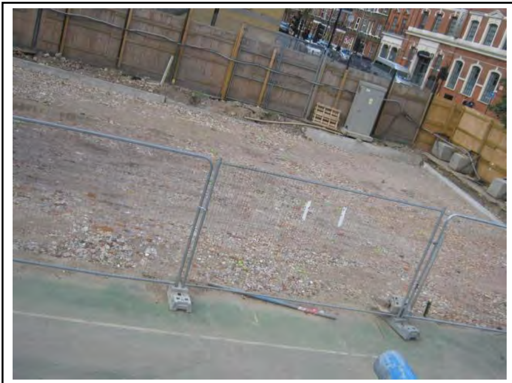
Installed piling mat.
