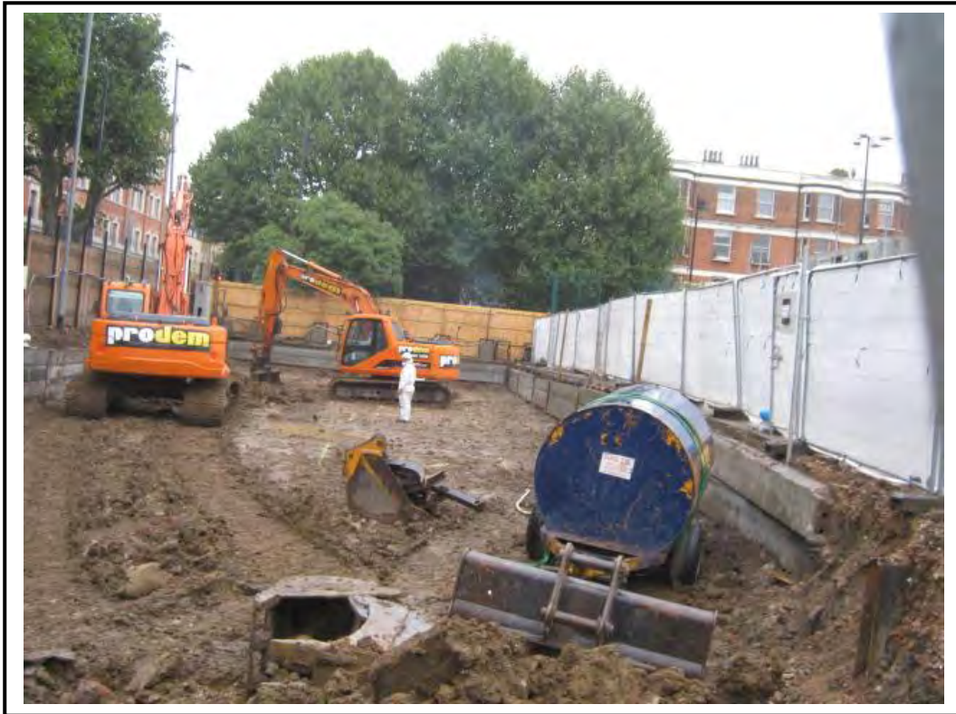
Excavation and damping down of asbestos contaminated soils.
