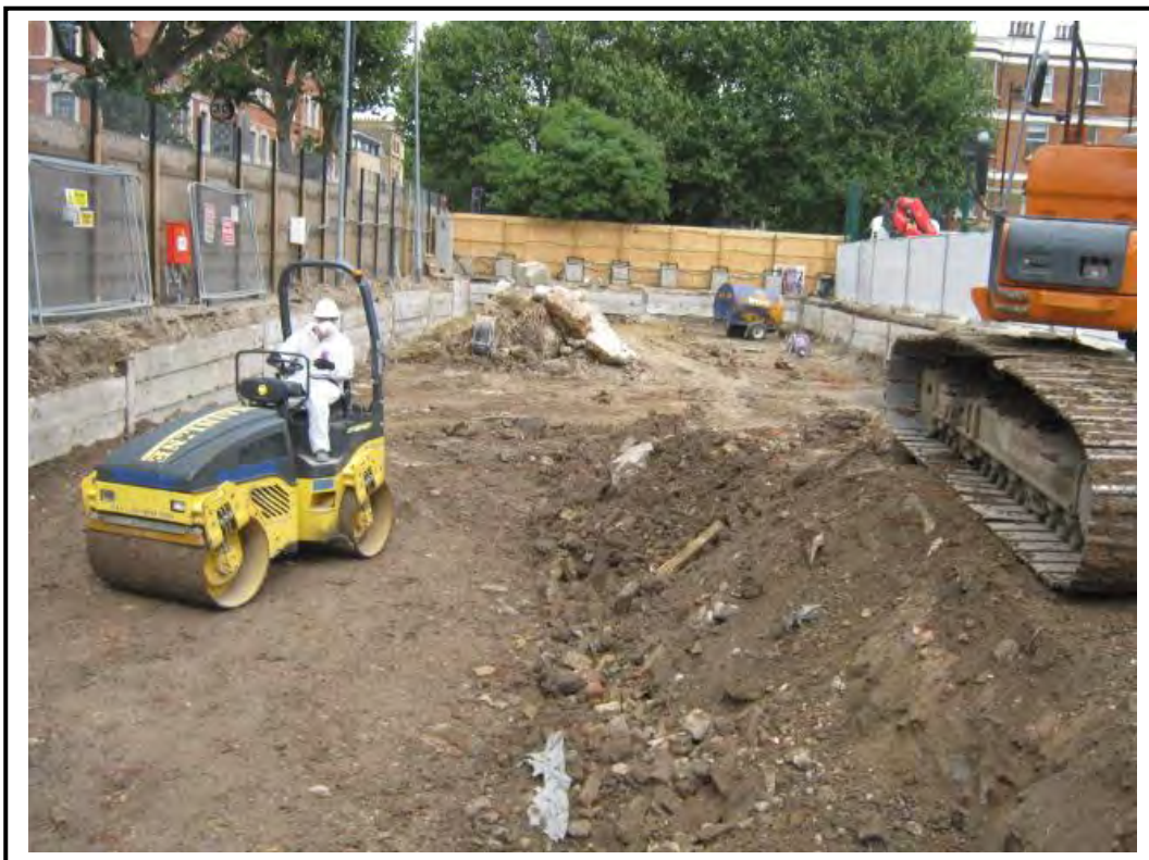
Placement of new soils.
