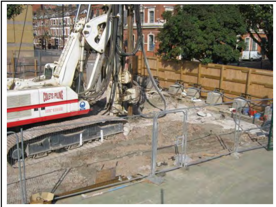
Piles installed across the eastern limb of the site.
