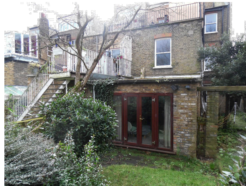
EXISTING REAR EXTENSION
