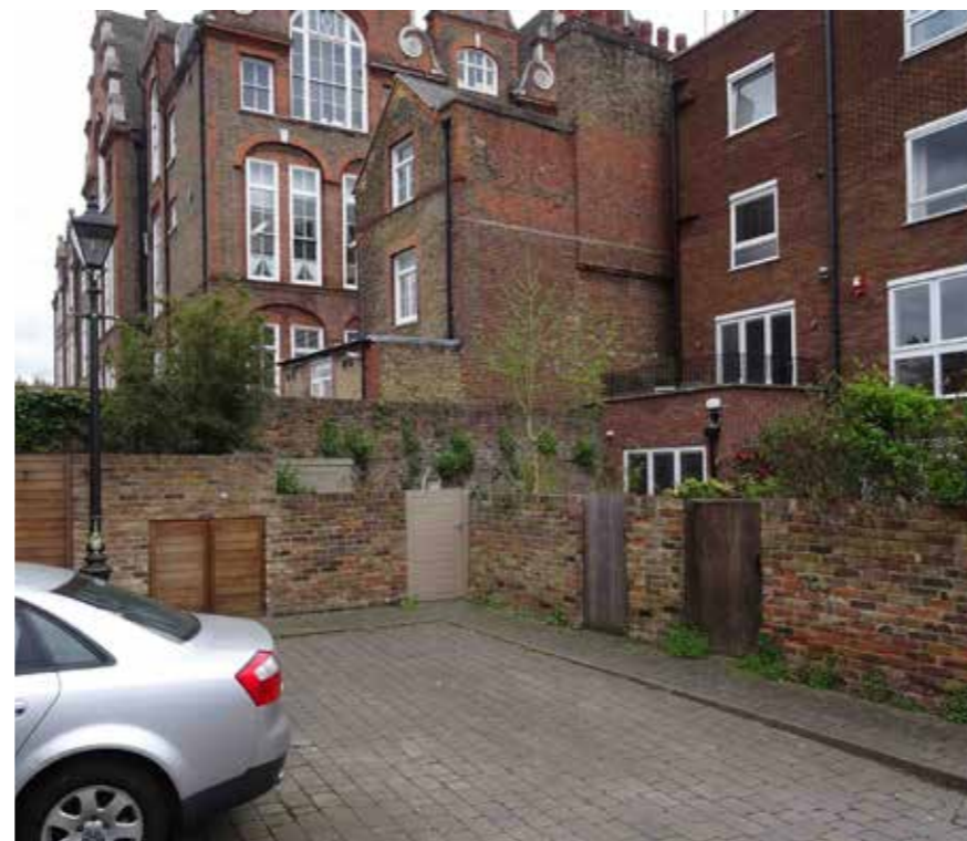
Fig 4.4 View from Waterside Place of the rear of no. 46 Princess Road and the north-east side of the Caretaker's house.
