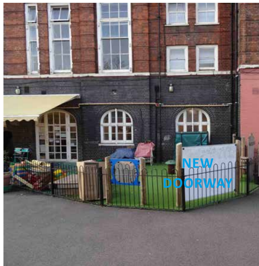
Recent example (2003) of window arch converted to doorway (left-hand door).
