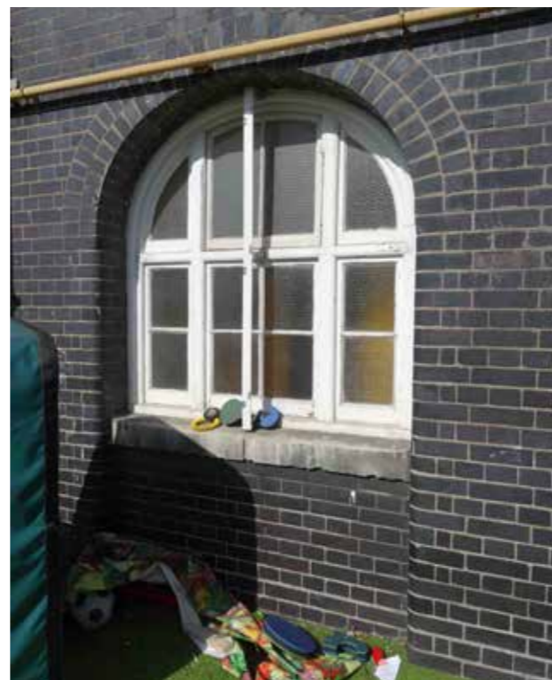
Fig 4.7 The original window to be converted to an open doorway.
