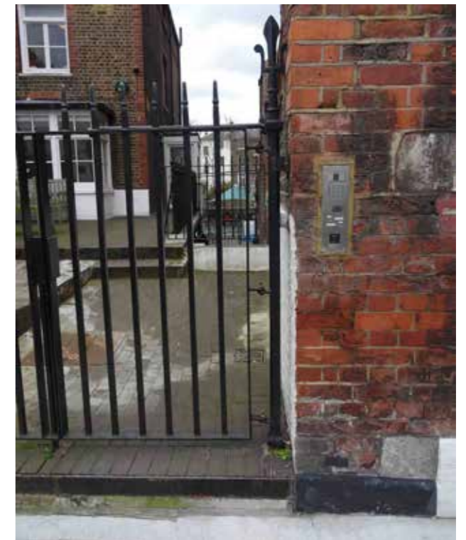
Fig 4.2 The step on the right-hand side is to be removed, and bars on the right-hand leaf extended down. The original post is to be retained.
