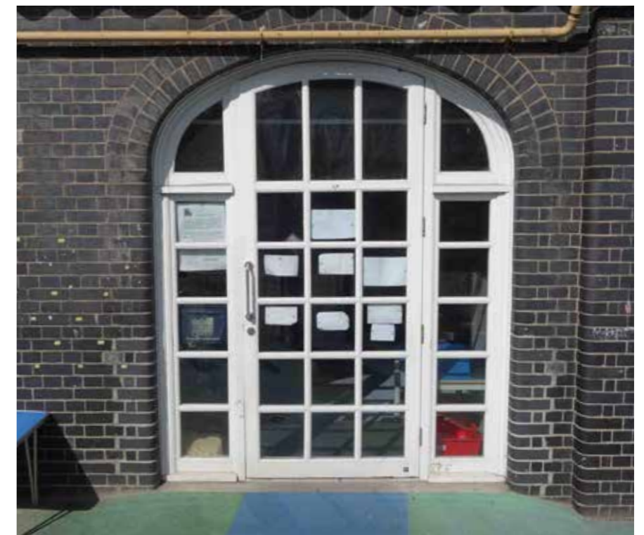
Fig 4.8 An adjacent dropped window converted to a door using Ibstock Atlas Smooth Blue bull-nosed bricks.
