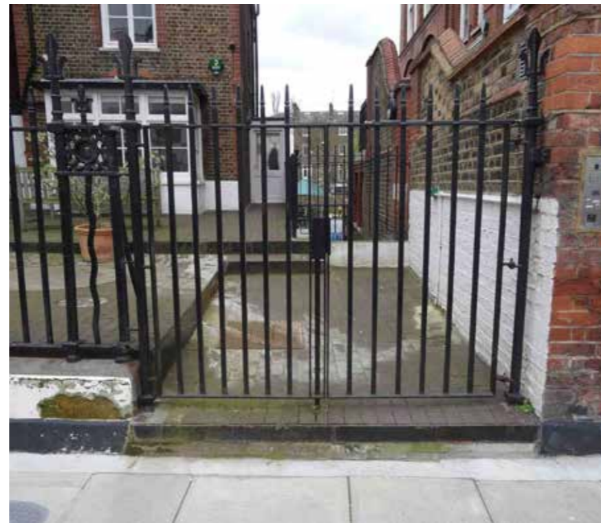
Fig 4.1 The stepped entrance and recent gate (2011) to the Caretaker's house.
