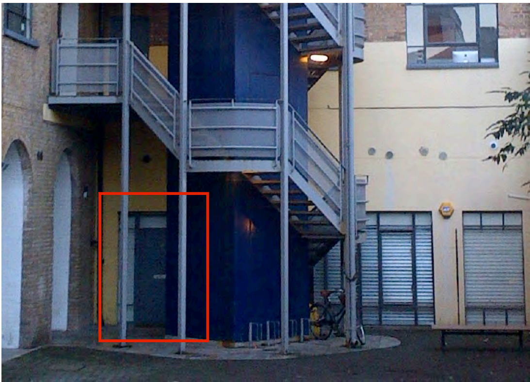
The door of Unit 7 on the ground floor will have to be relocated withouth side glazing to allow new lift shaft against the wall (see drawing AS-ST pr 8)
