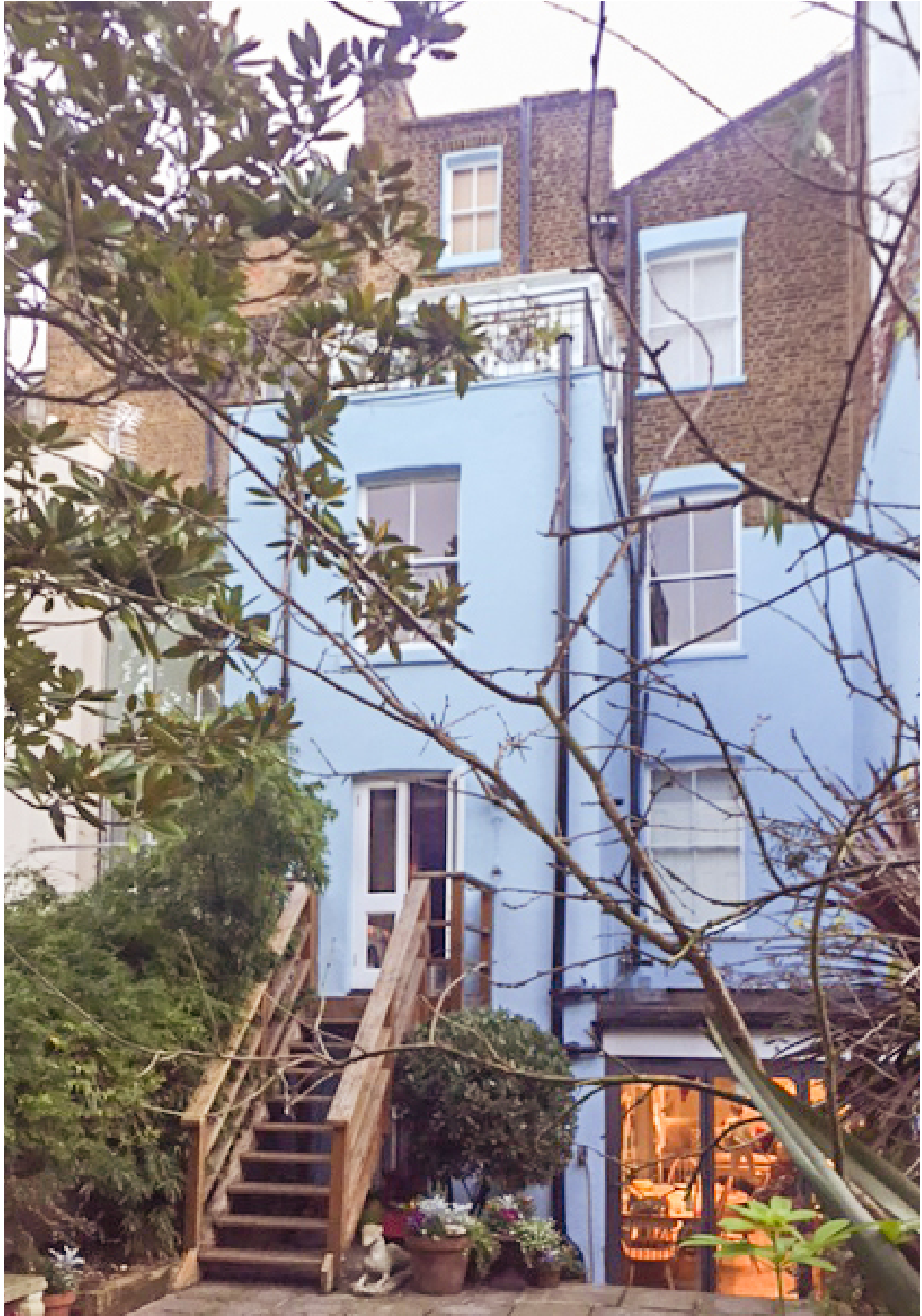
171 Gloucester Avenue Rear Elevation (South West)
