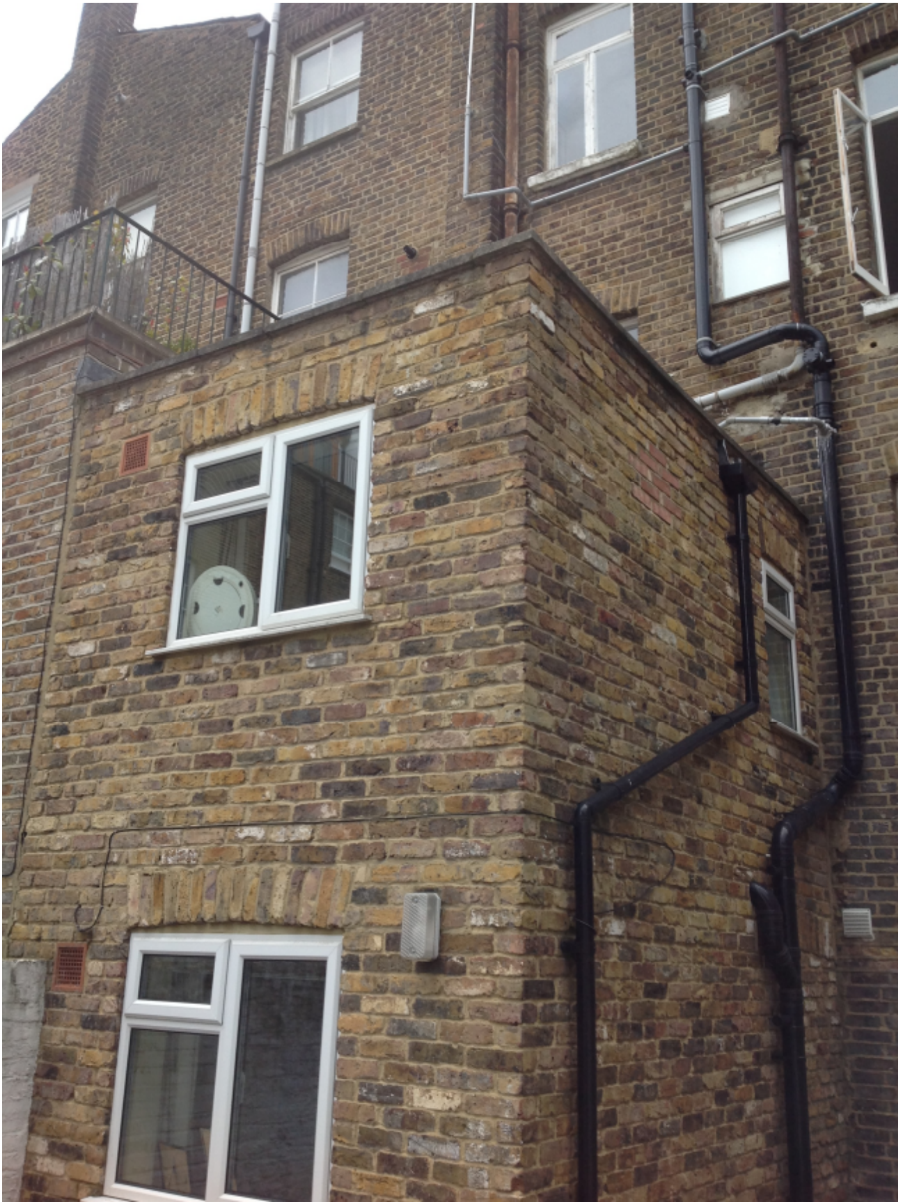
Photo 4: View of existing flat roof from rear courtyard of 44 Chalcot Road
