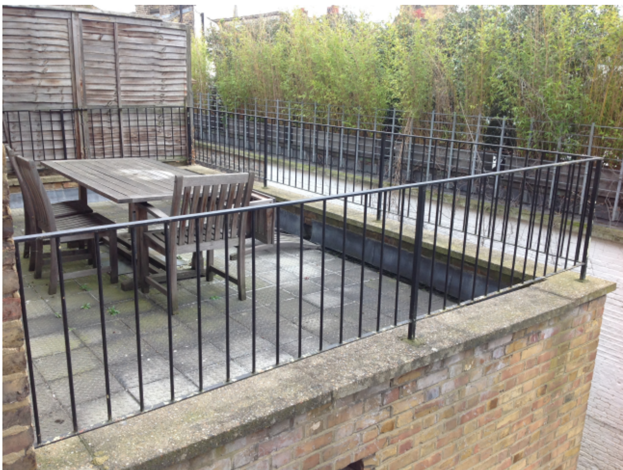
Photo 6: Neighbouring terrace at no. 45 Chalcot Square
