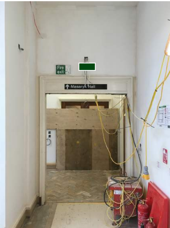
Above Door wall mounted
