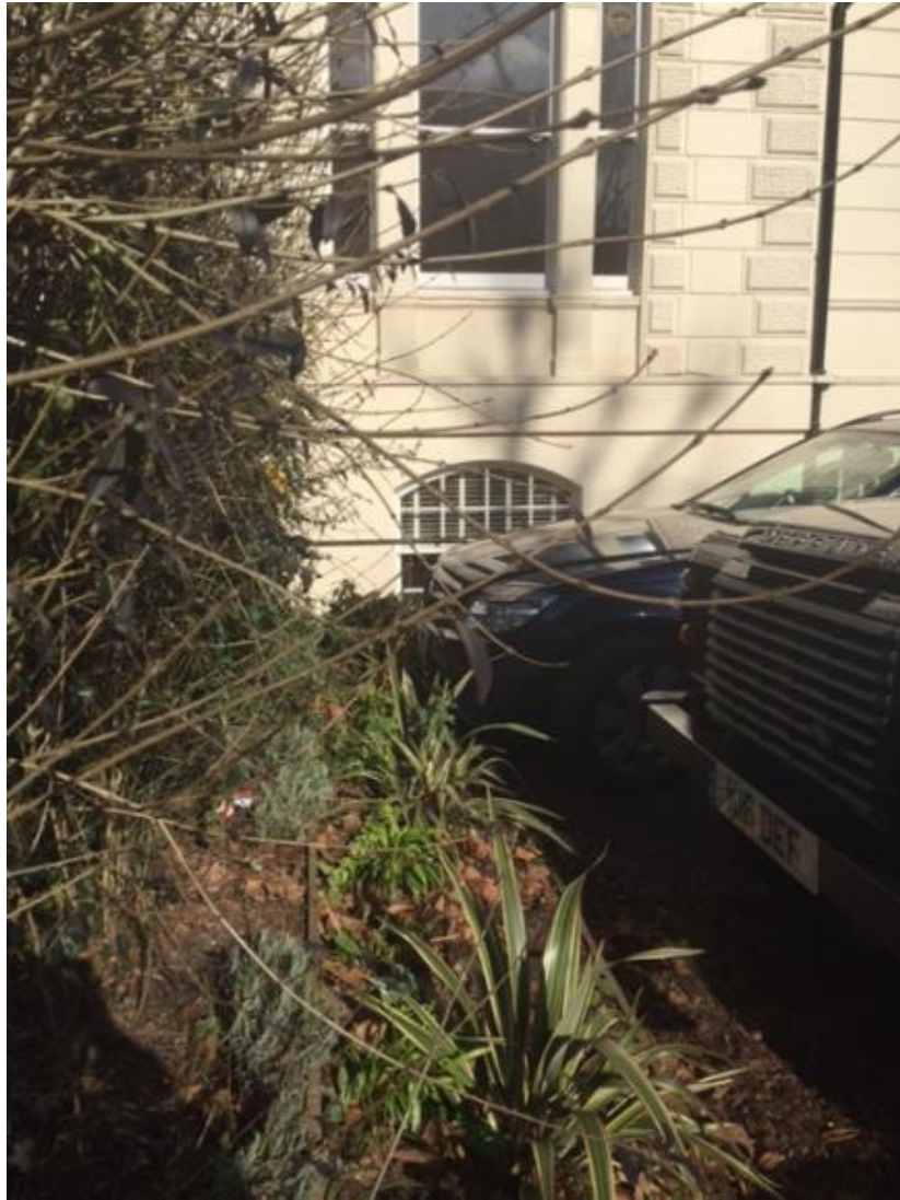
Photo 2 – View of window from the driveway
