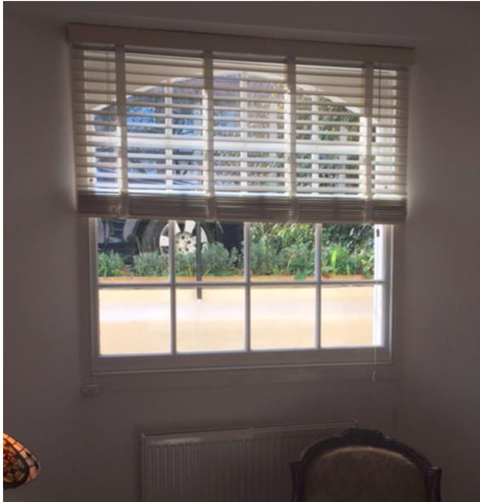
Photo 5 – Window from inside the property
