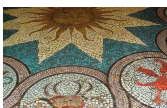
Existing Details - Staircase Balustrade & Lobby Floor
