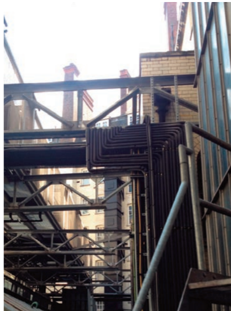
Existing Lift Shaft, Plant Cage & Services
