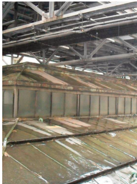
Existing Lantern Roof & Plant Cage
