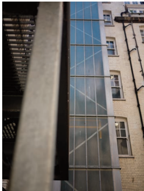
Existing Lift Shaft - Georgian Wired Structure
