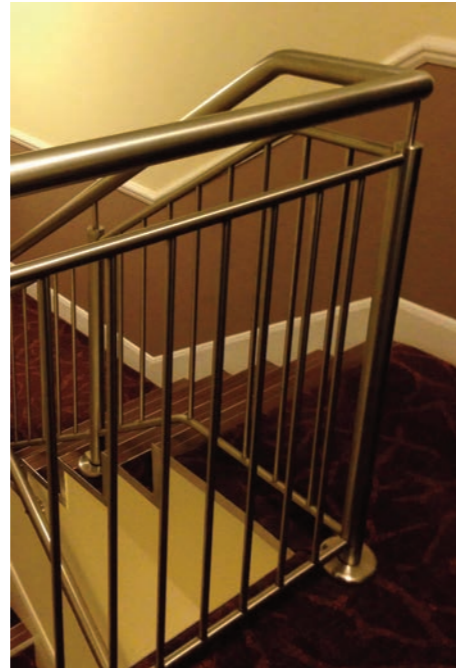
Existing Dog-leg Stair under Feature Staircase
