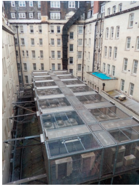
Existing Lightwell with Plant Cage
