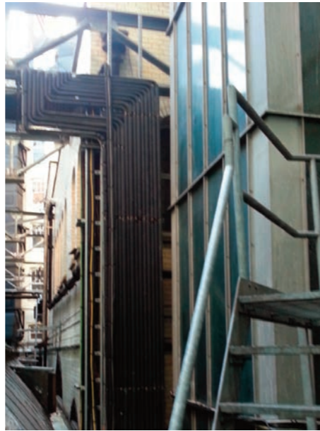
Existing Lift Shaft, Services & Plant Support
