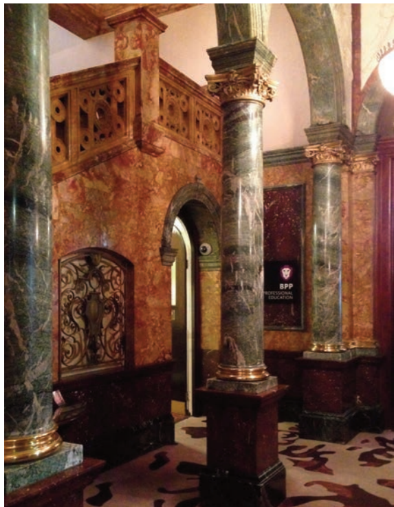
Existing Lobby - view into doorway to lower ground stairwell
