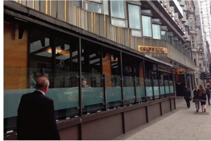
The Imperial Hotel, External Seating Area
