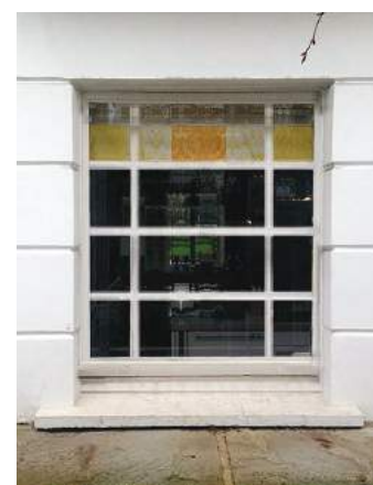
Fig 20 & 21 _ Proposal to remove security bars and replace existing single glazed window with thermally broken steel window
