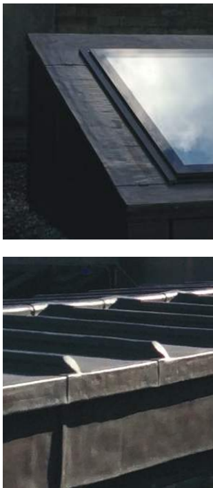
Fig 14 _ Examples of lead flashing
