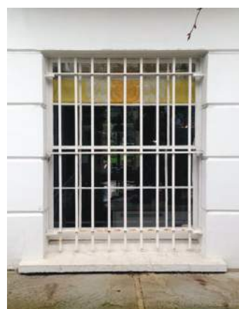
Fig 20 & 21 _ Proposal to remove security bars and replace existing single glazed window with thermally broken steel window
