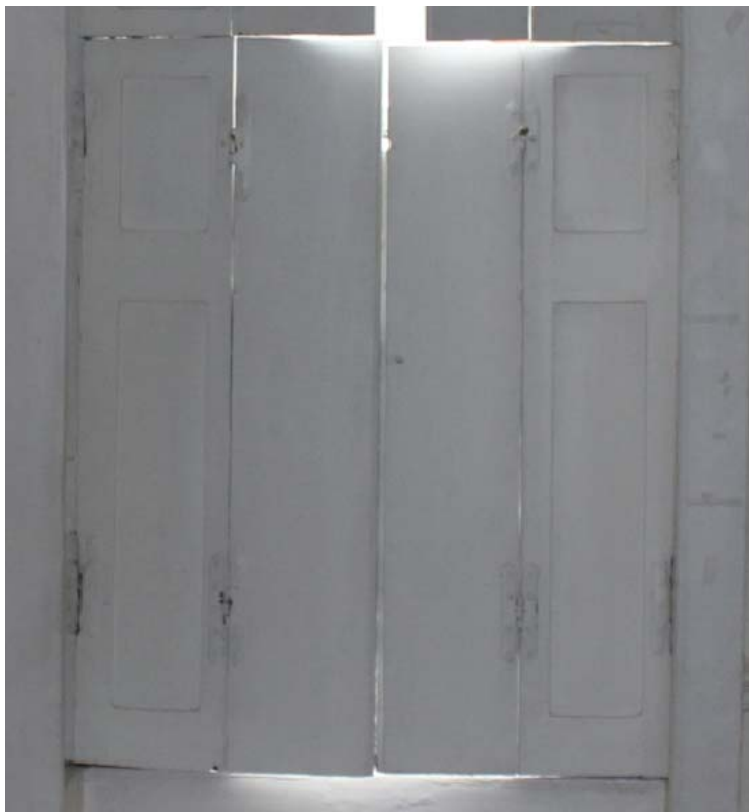
Existing window shutters showing long 'H' profile hinges
