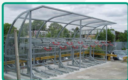
Solent extended shelter (Upminster station)
