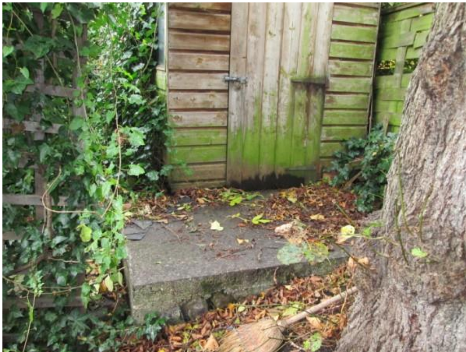
Existing shed and concrete base
