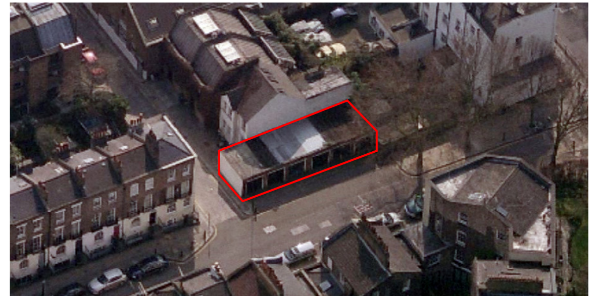
Aerial view from the north (Courtesy Bing Live Maps)
