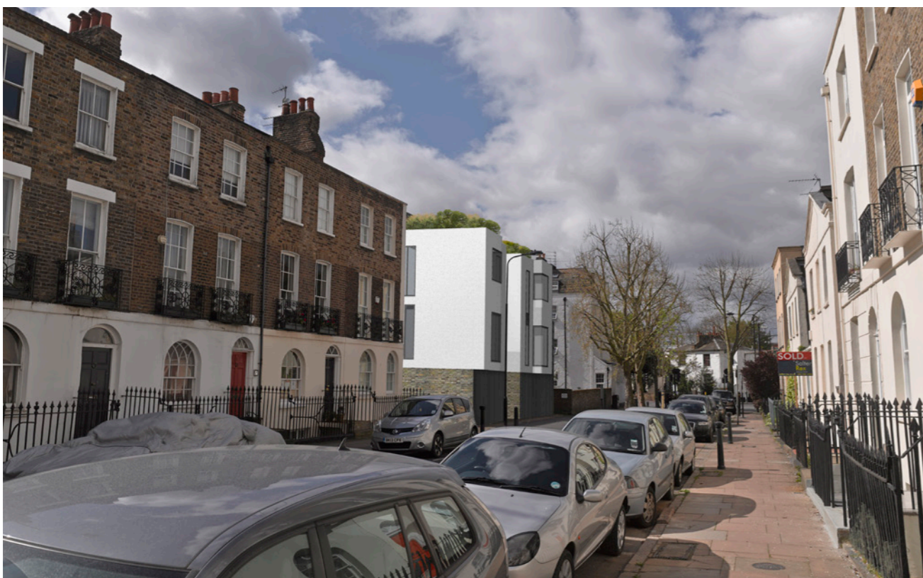
03- Emrys Architects existing planning permission - Jeffrey's Street view 02
