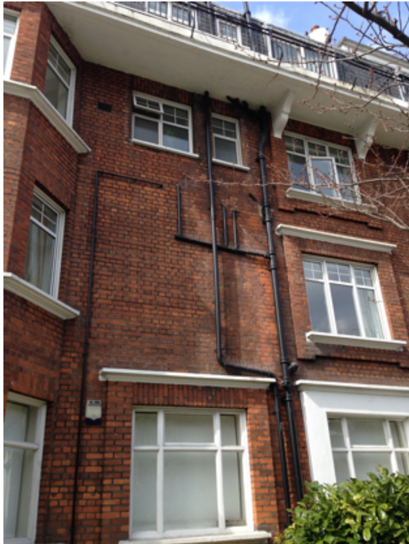
Figure 3, 1 Fortune Green Road depicts the use of external SVP on the main elevation of the building.
