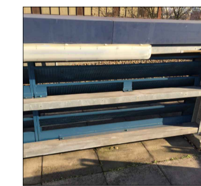
PHOTO 3 - VIEW OF EXISTING INTERNAL FACE OF LOUVERED WALL.
