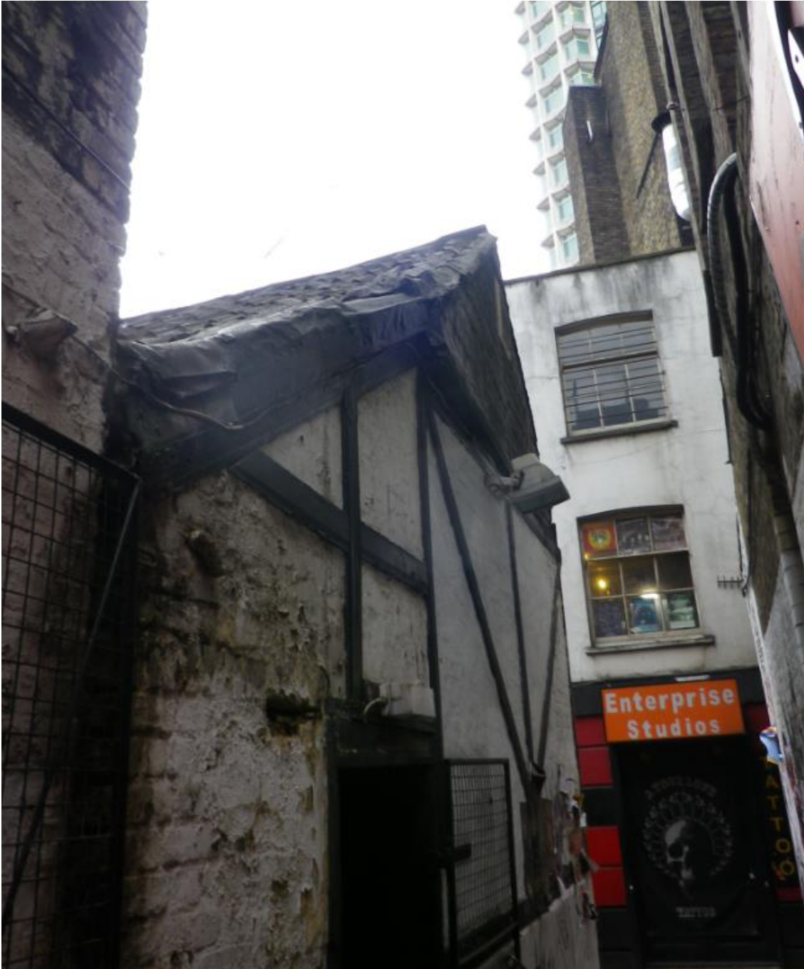
Above: 22 Denmark Place (The Smithy)
