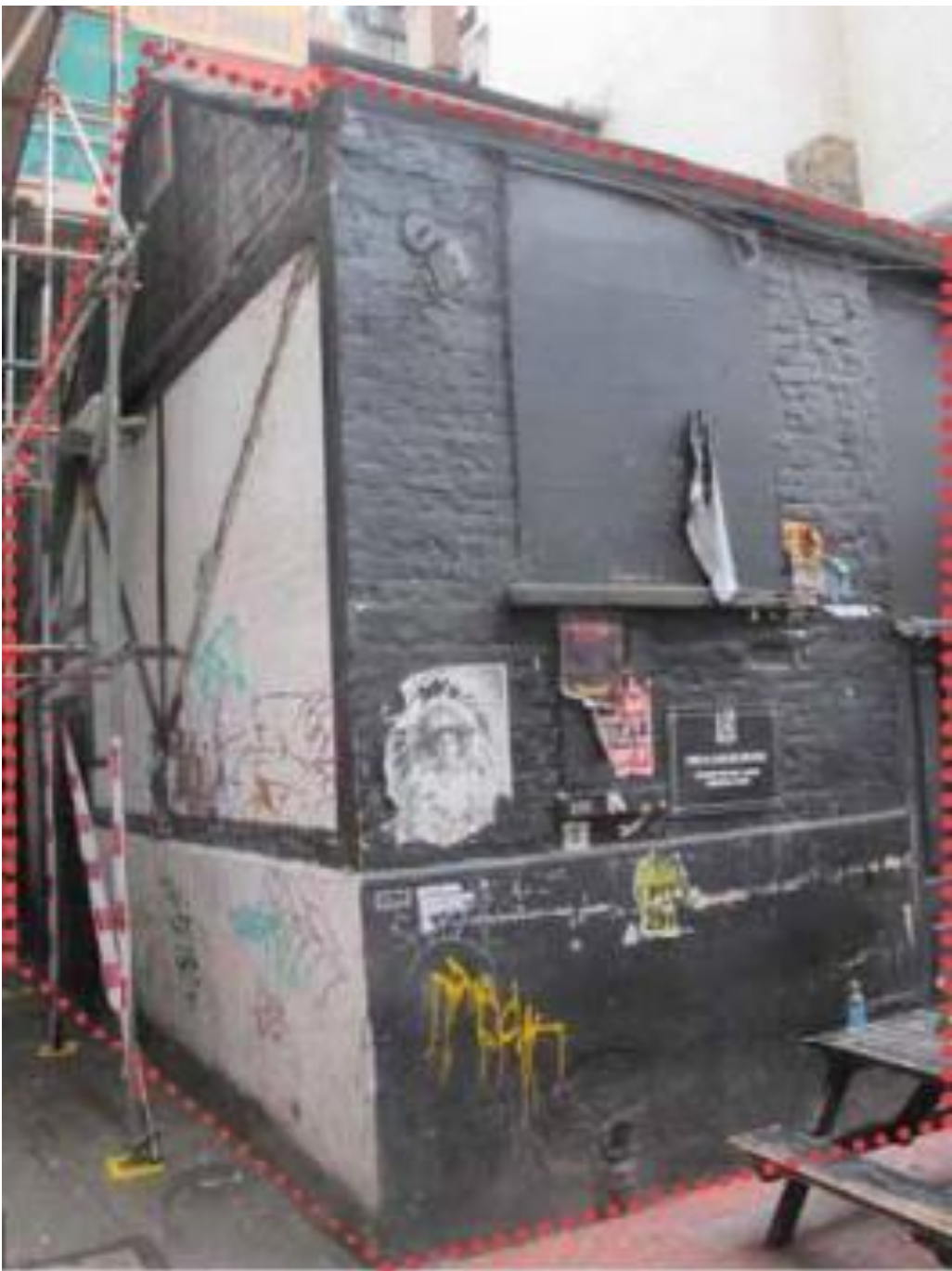
Above: 22 Denmark Place (The Smithy)
