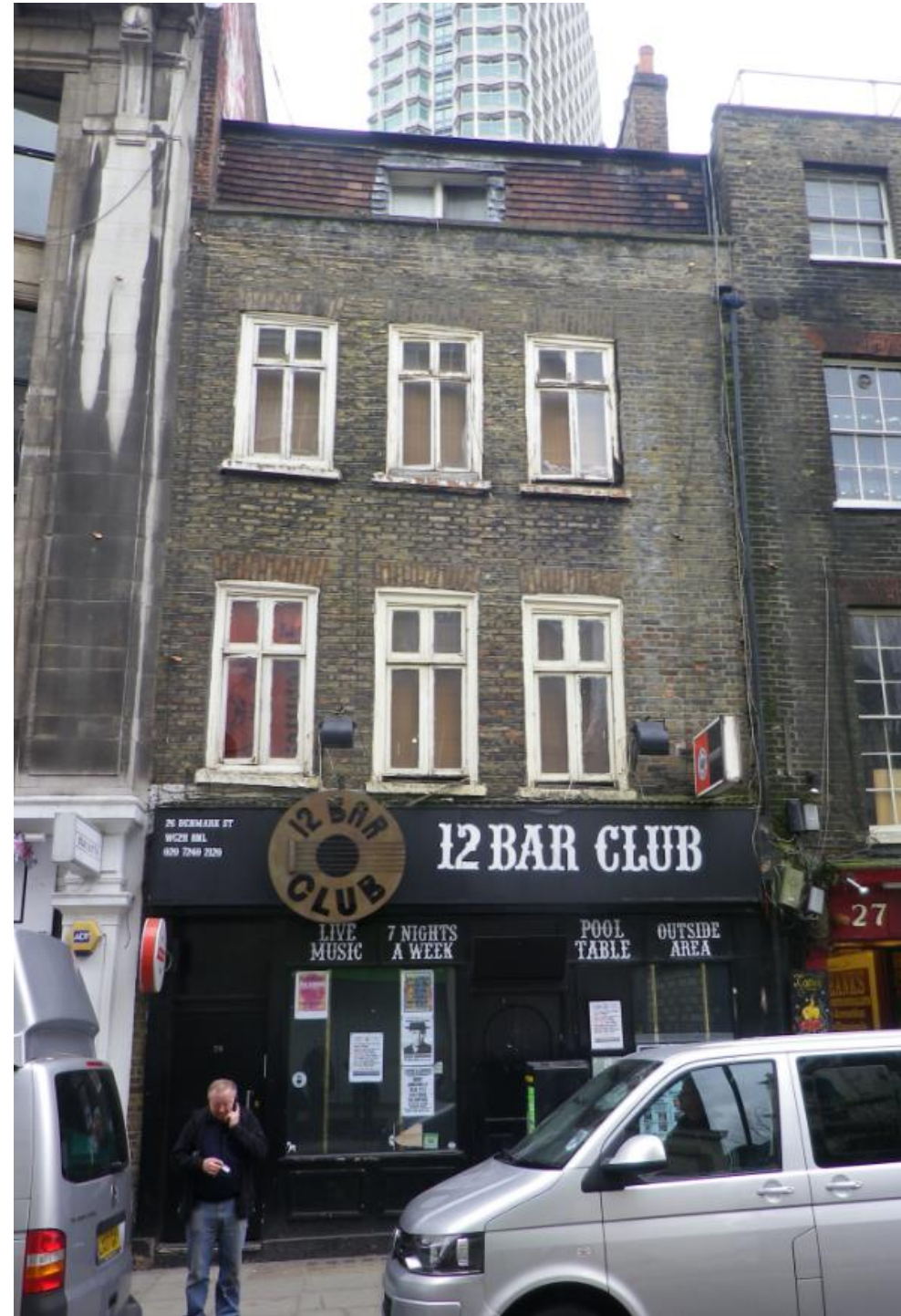
Above: Front elevation of 26 Denmark Street
