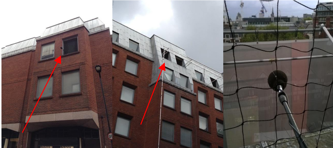
Figure 3 Photograph showing location of L1, L3 and the view from L2
