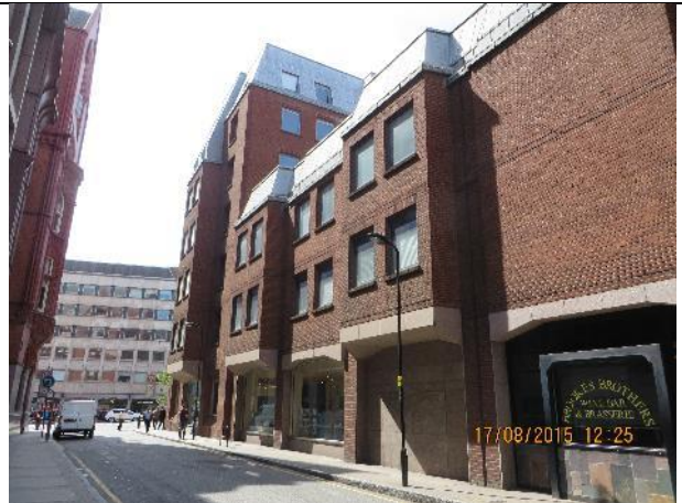
Photograph 2: Eastern elevation of 150 Holborn
