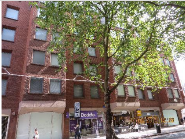
Photograph 3: Western elevation of 150 Holborn
