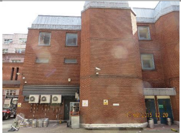
Photograph 4: Within the central courtyard of 150 Holborn
