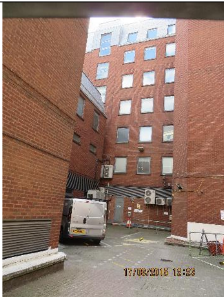
Photograph 5: Within the Site courtyard
