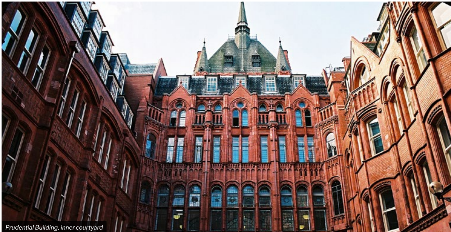
Prudential Building, looking east along Holborn
